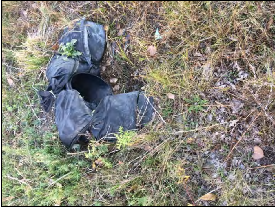
Control Structure (pipe with sandbags) at SW-1 (IMG_2247)
