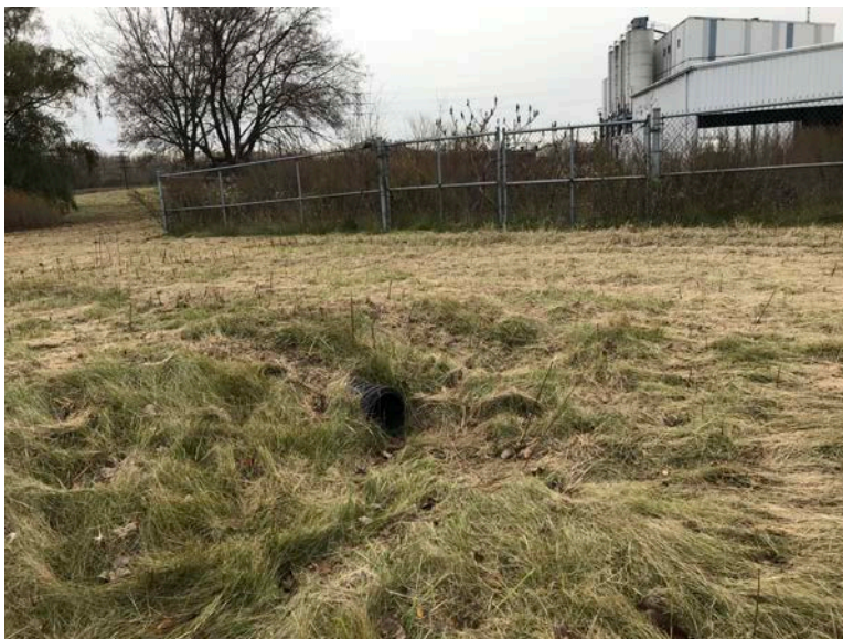
Storm water drainage system no standing water
