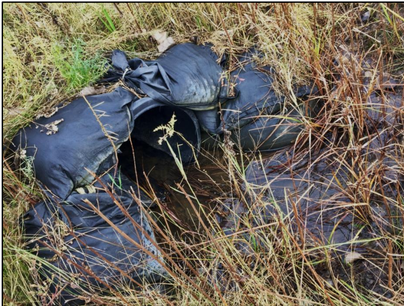
Culvert with sand bags (SW-1)
