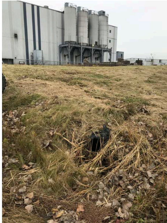
Culvert with sand bags (SW-1)
