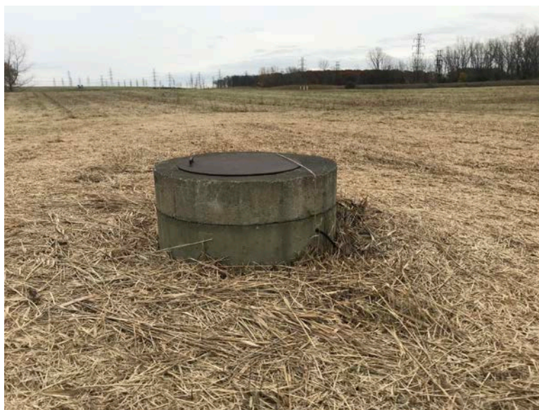
Sump Collection Tank (LS-1)
