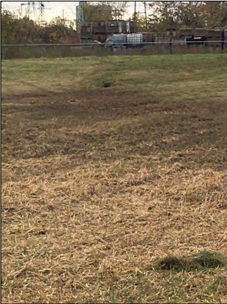
Culvert inlet and drainage swale
