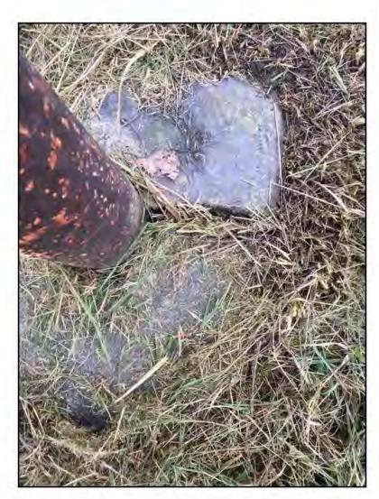
MW BR-1 broken pad, needs to be repaired
