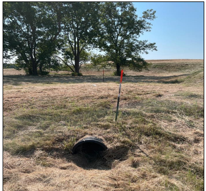
Culverts Connecting The Stormwater System
