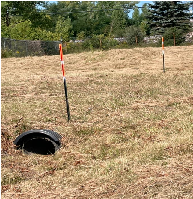
Culverts Connecting The Stormwater System
