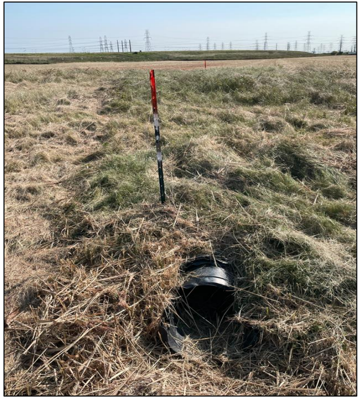
Culverts Connecting The Stormwater System
