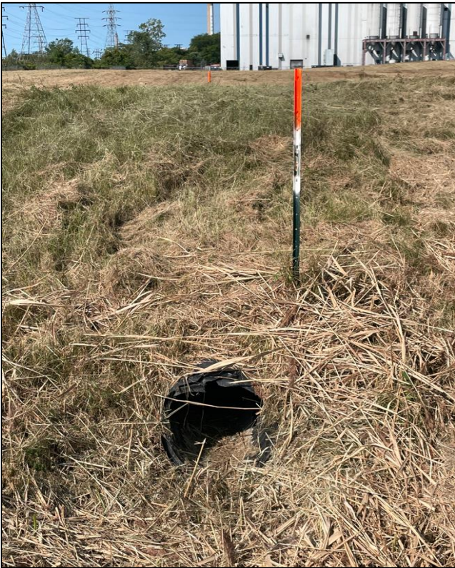
Culverts Connecting The Stormwater System
