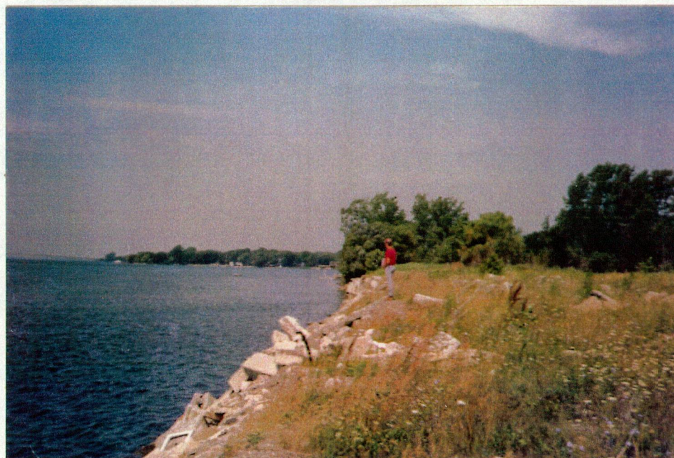
PHOTO 6. Concrete rubble breakwall on southern end of site, looking west.
