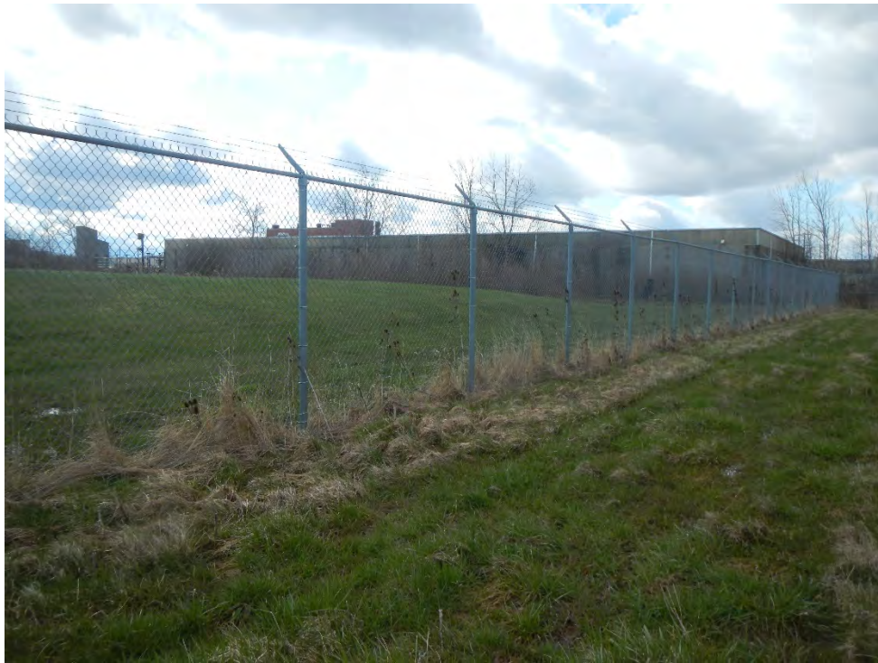
Photo 3 - View of west side of cap viewed from NFTA property
