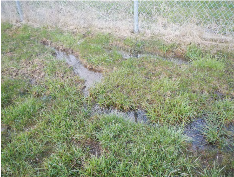
Photo 15 - View of west side of cap (southern end) and ruts from lawnmower
