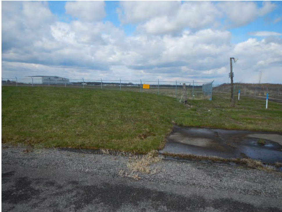
Photo 9 - View of north side of cap
