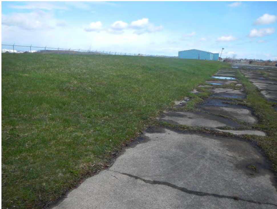
Photo 20 - View of east side of cap
