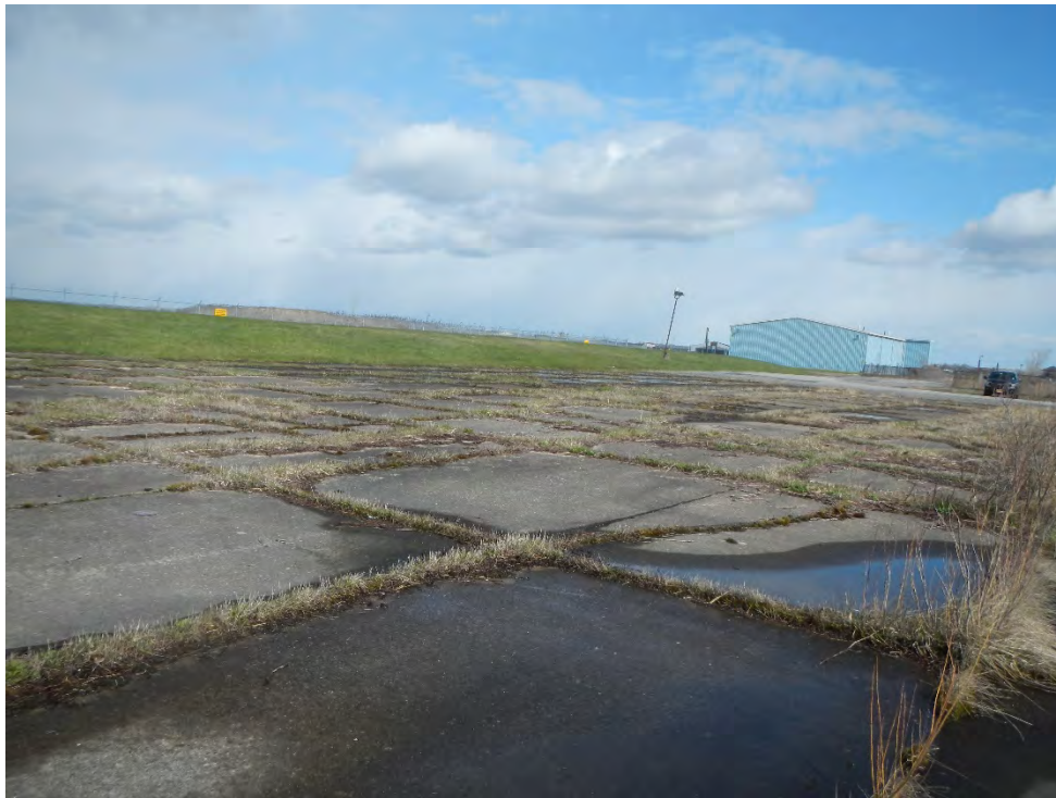
Photo 22 - View of east side of cap
