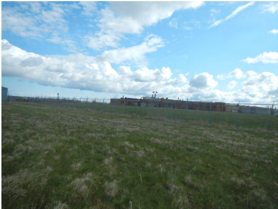
Photo 6 - View of west side of cap viewed from NFTA property
