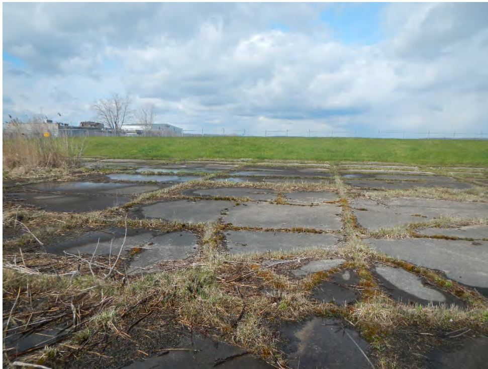
Photo 23 - View of east side of cap
