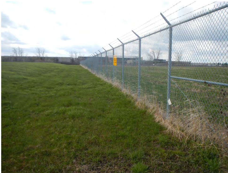
Photo 13 - View of west side of cap
