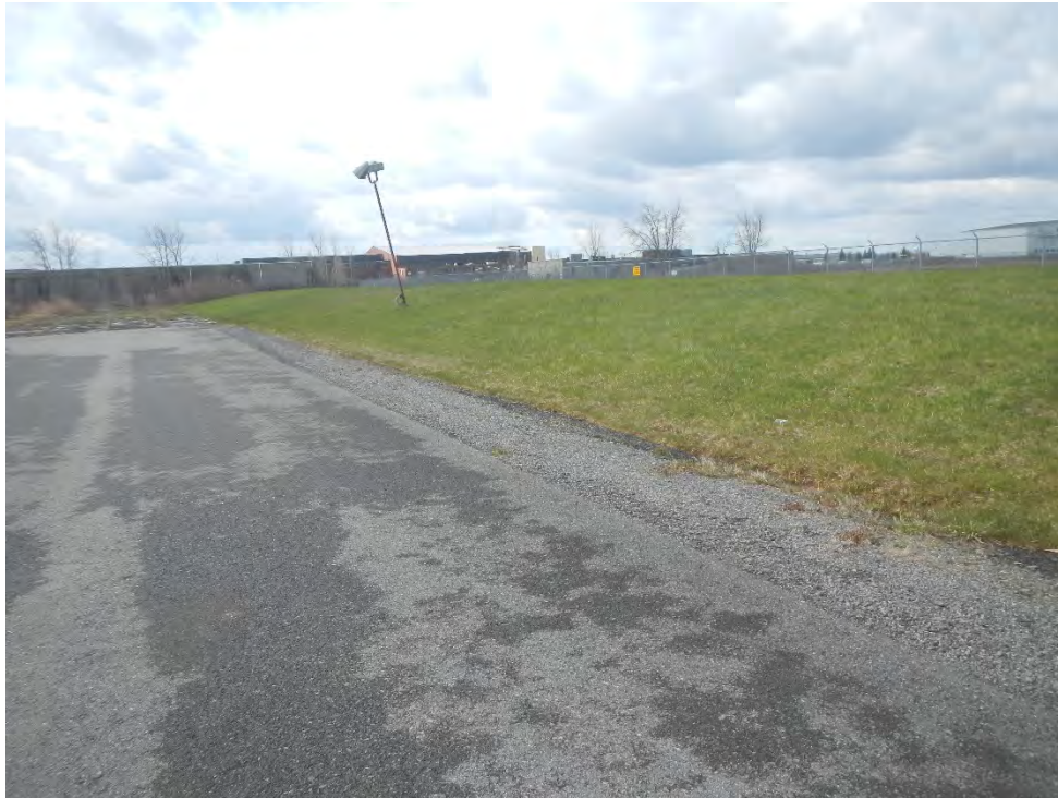
Photo 10 - View of east side of cap
