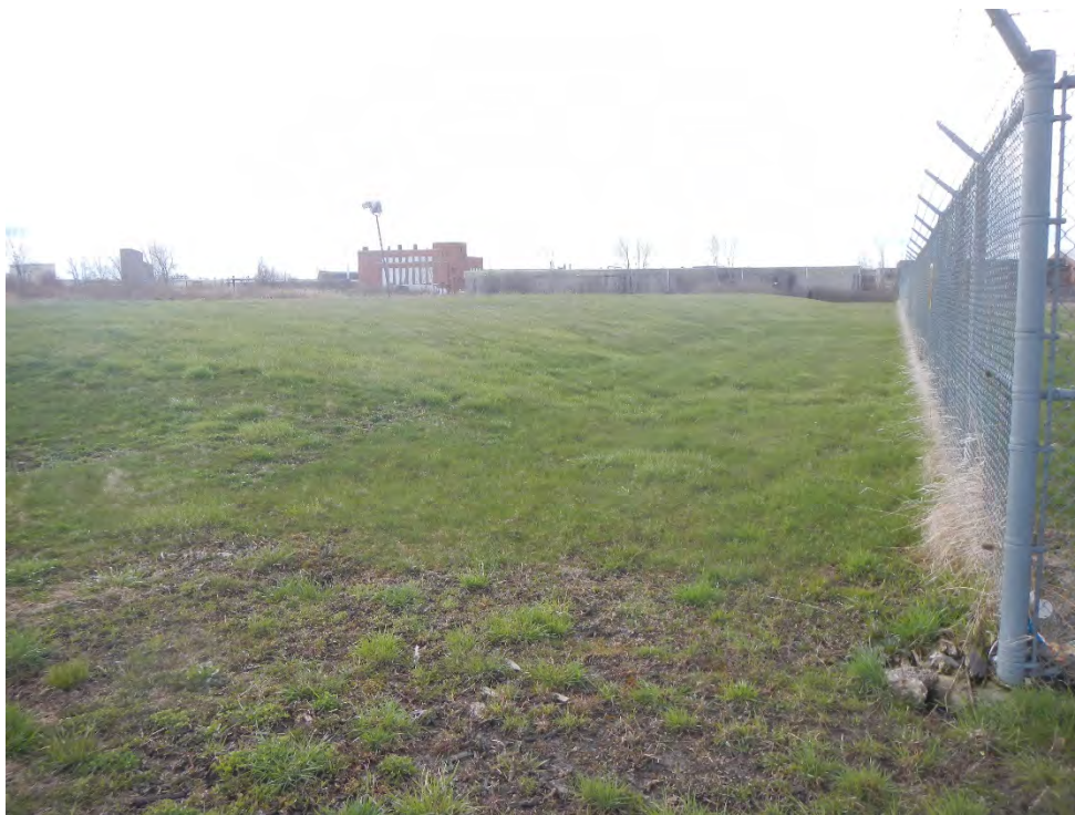
Photo 11 - View of west side of cap as viewed from the Site
