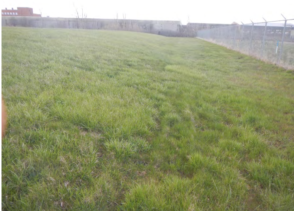
Photo 14 - View of west side of cap
