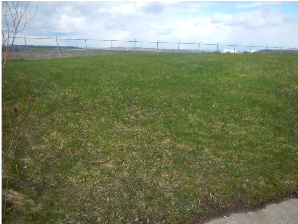
Photo 19 - View of south side of cap
