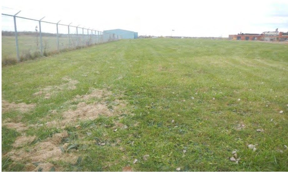
Photo 3 View of west side of cap facing north
