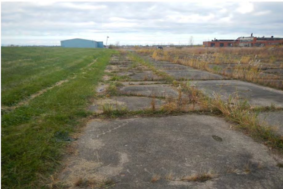
Photo 22 View of concrete area east of Site with monitoring wells
