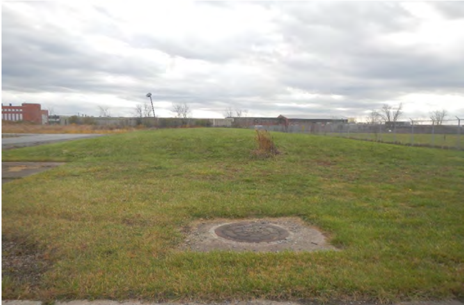
Photo 10 View of north side of cap
