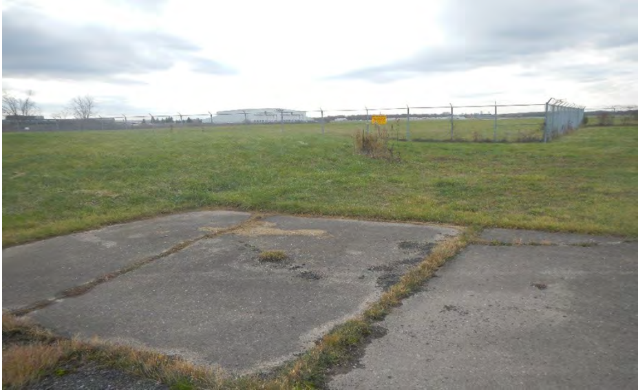
Photo 11 View of north side of cap
