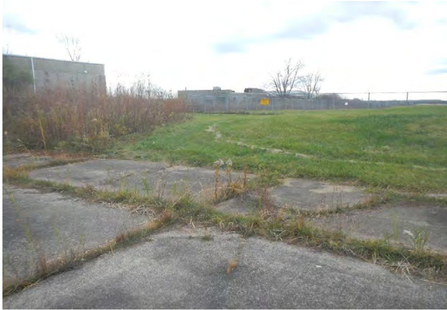
Photo 13 View of east side of cap
