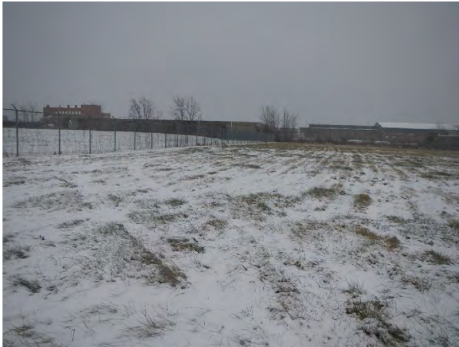
Photo 26 View of west side of cap viewed from NFTA property
