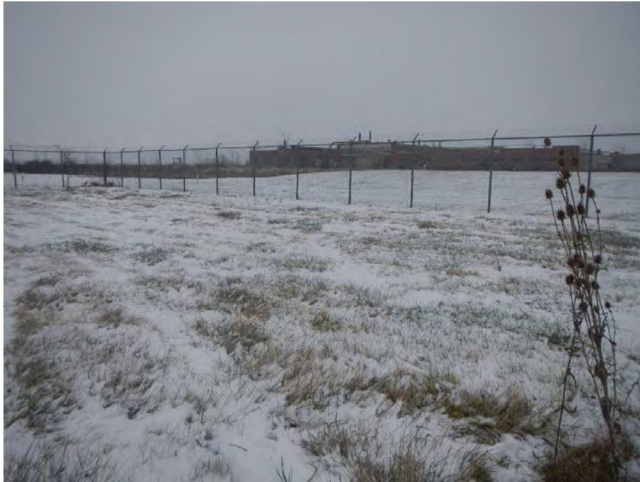
Photo 25 View of west side of cap viewed from NFTA property
