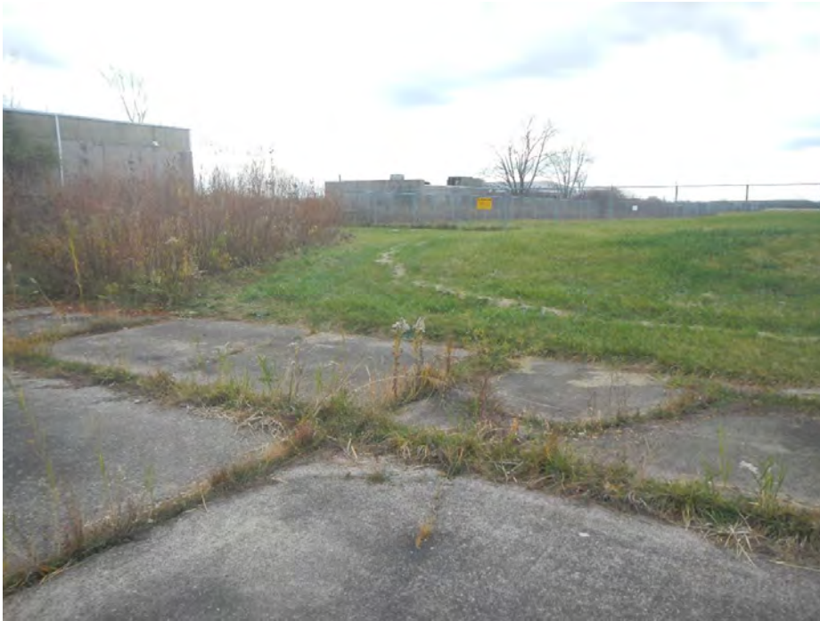
Photo 1 View of south side of cap
