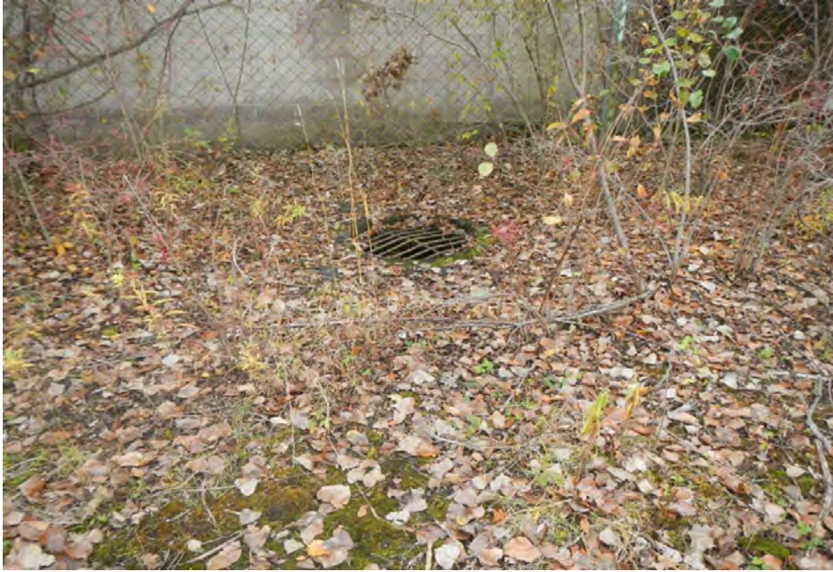
Photo 17 View of un-numbered manhole/catch basin
