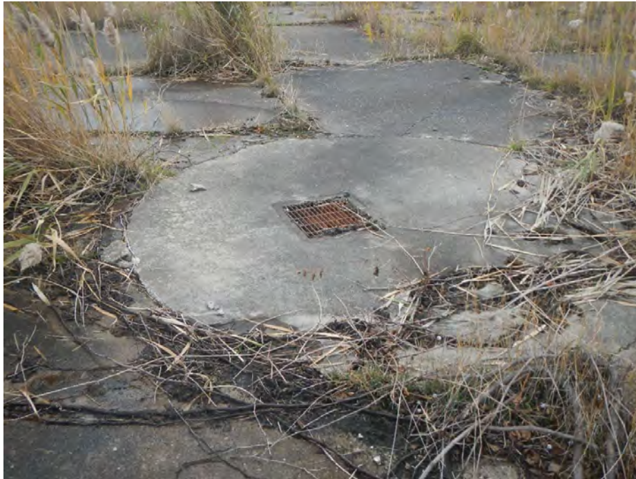
Photo 19 View of MH A-10 east of Site
