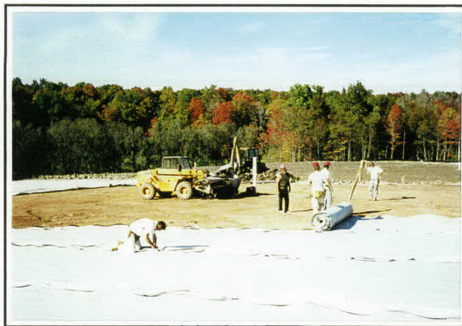
Photo #14: Geocomposite Installation
