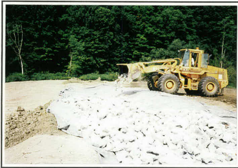
Photo #21: Rip-Rap Placement in Downchute
