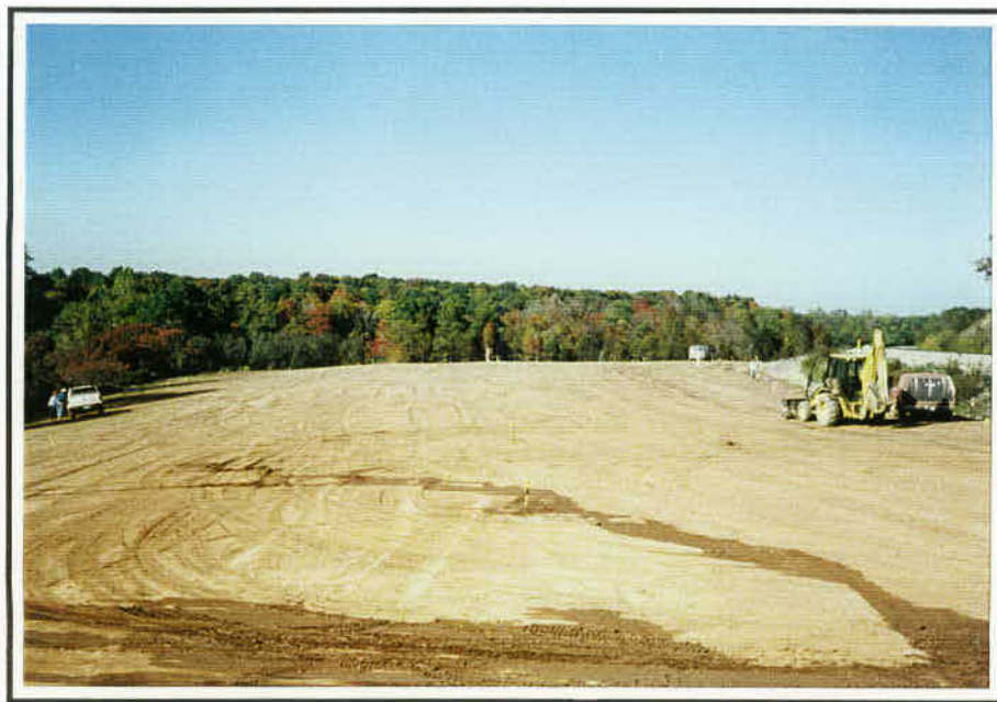
Photo #12: Subgrade Preparation
