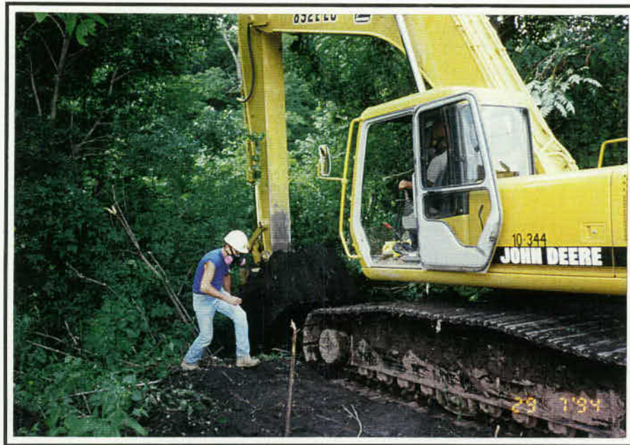
Photo #5: Test Pit Excavation on the "Very Steep" Slope
