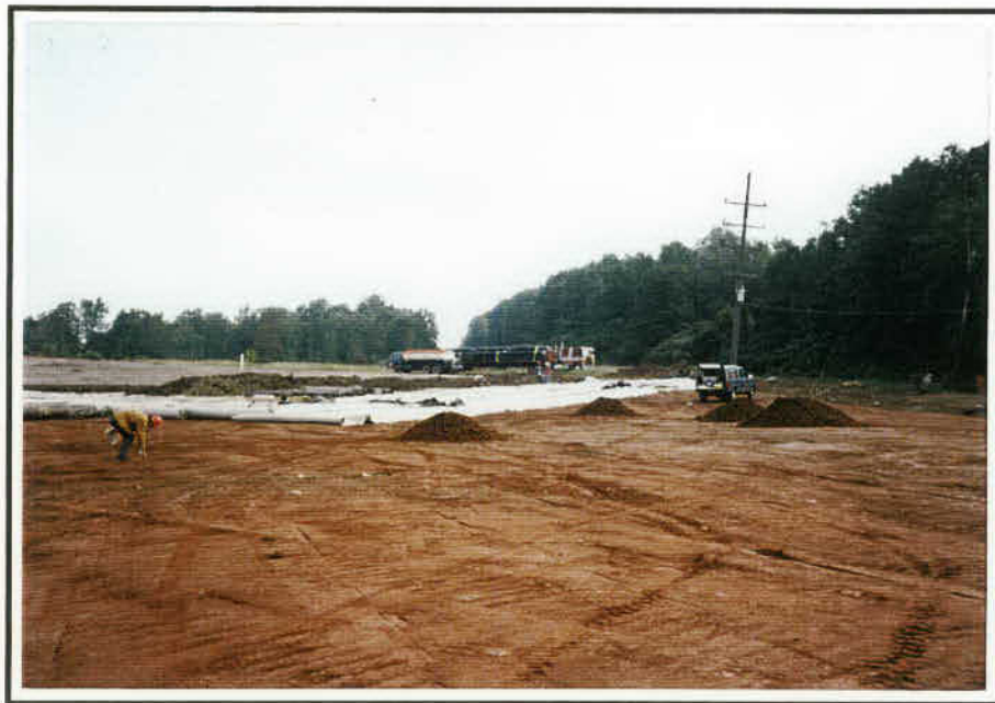
Photo #11: Subgrade Preparation, Geocomposite Installation, and LPS Layer Construction
