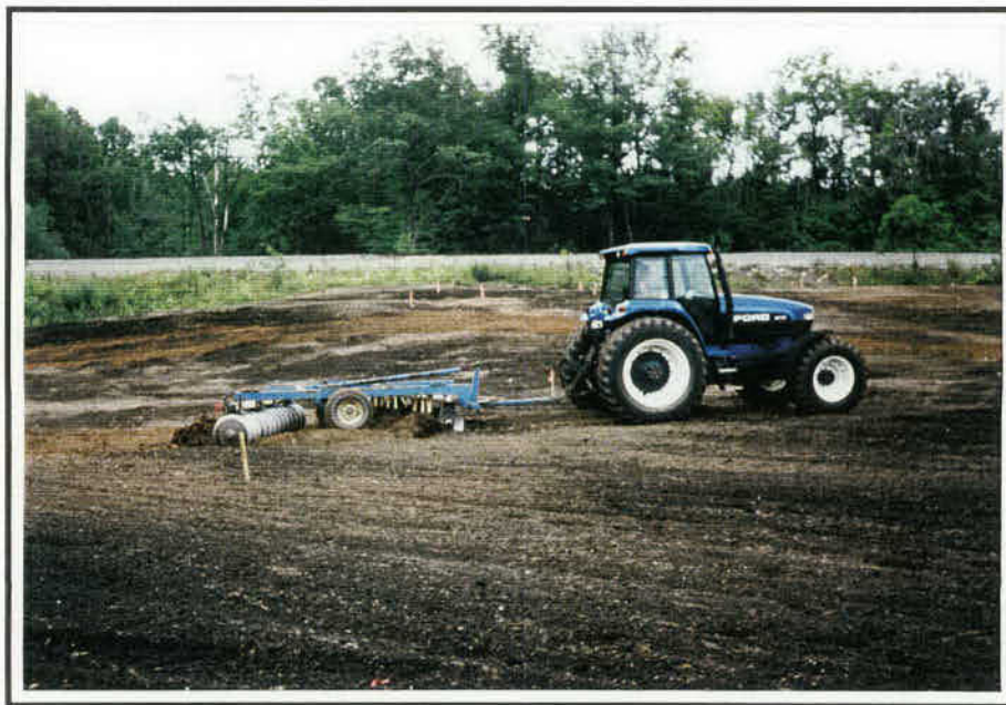
Photo #24: Compost/Soil Blending for Topsoil
