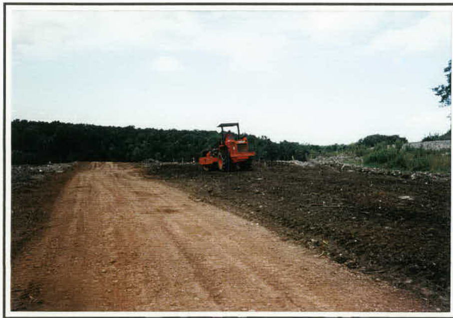
Photo #10: Relocated Waste Compaction
