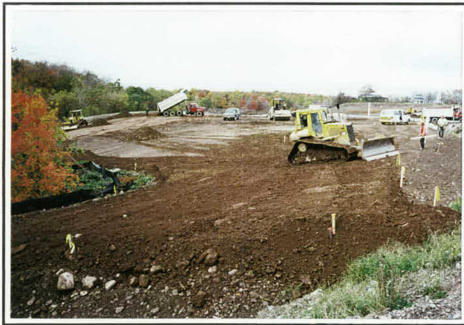
Photo #20: Barrier Protection Layer Placement - 2nd Lift
