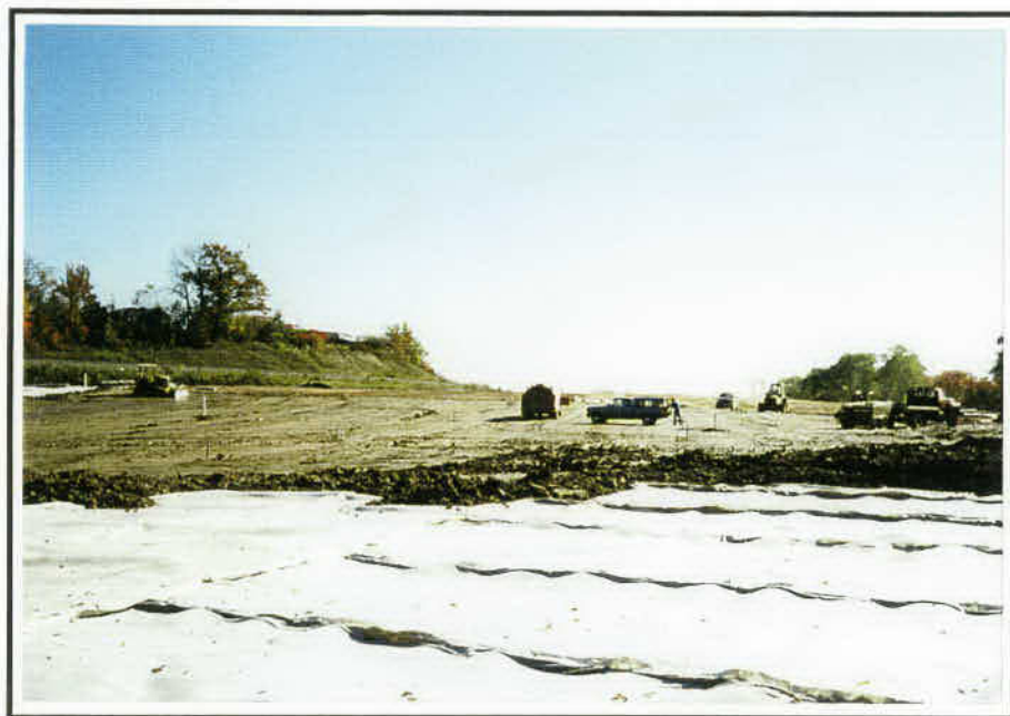
Photo #13: Geocomposite Installation and LPS Layer Construction
