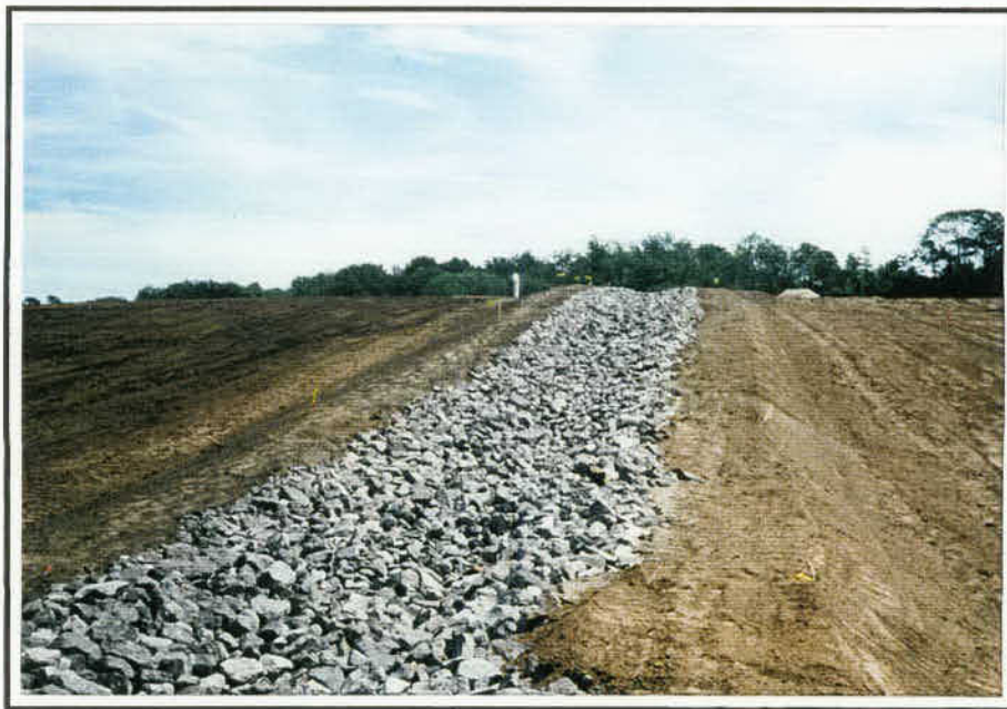
Photo #22: Completed Downchute
