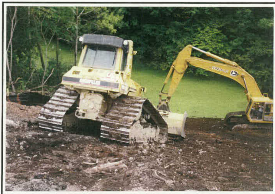
Photo #7: Grading and Excavation of the 1V on 2H Slope (Very Steep Slope)
