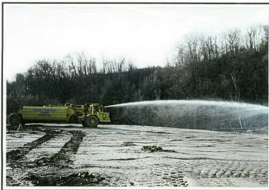
Photo #18: Moisture Maintenance of the LPS Layer
