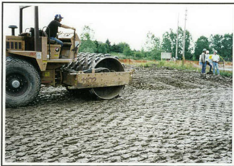
Photo #17: Compaction of the LPS Layer
