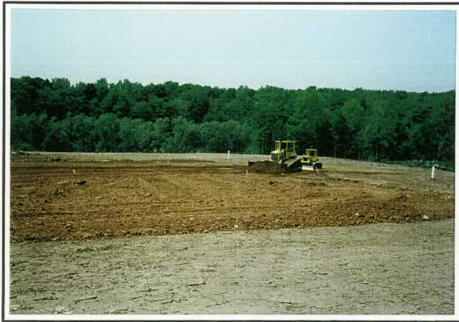
Photo #19: Barrier Protection Layer Placement - 1st Lift
