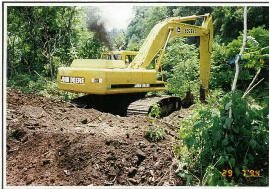
Photo #6: Excavation of the 1V on 2H Slope (Very Steep Slope)
