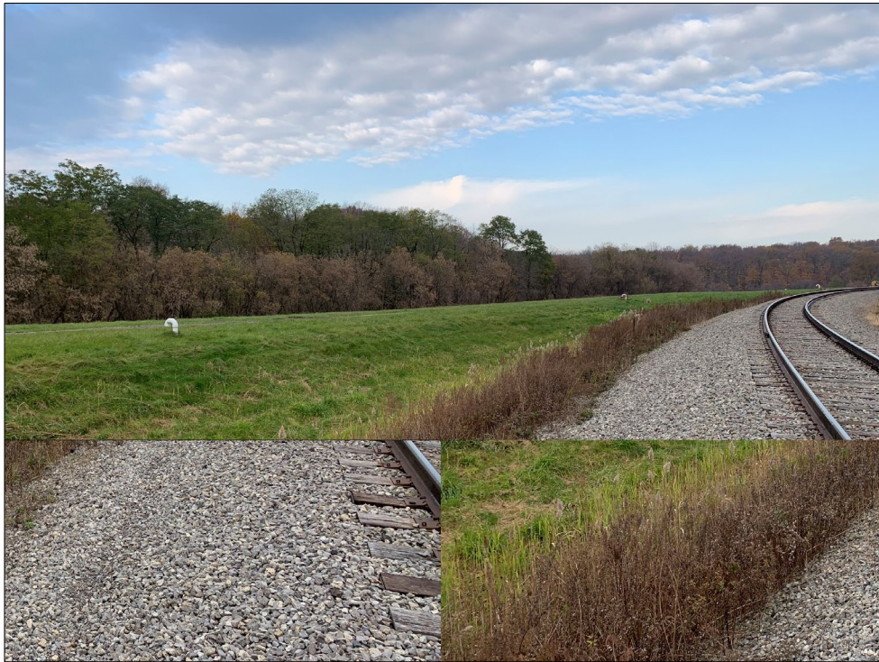
Photo 8 Site facing northwest across Drainage Ditch C
