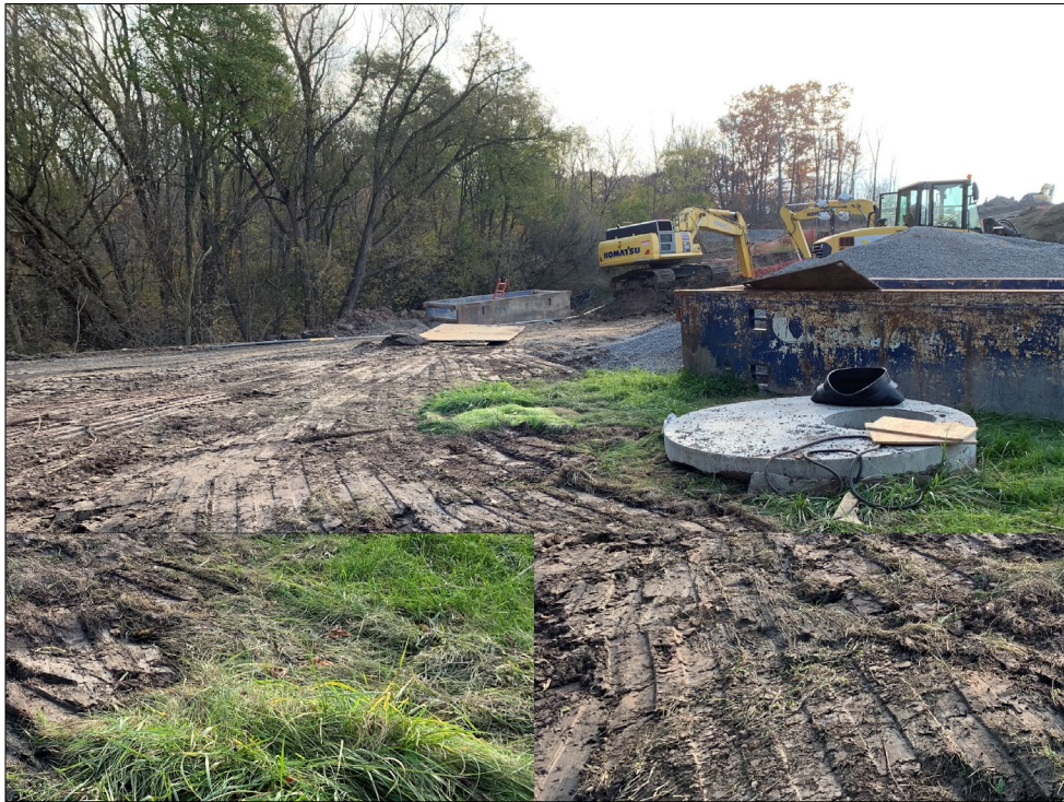
Photo 4 Construction area in northeast corner facing southeast
