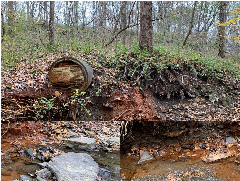
Photo 6 Outfall L-2, with seep and exposed trash to the right of the outfall along bank
