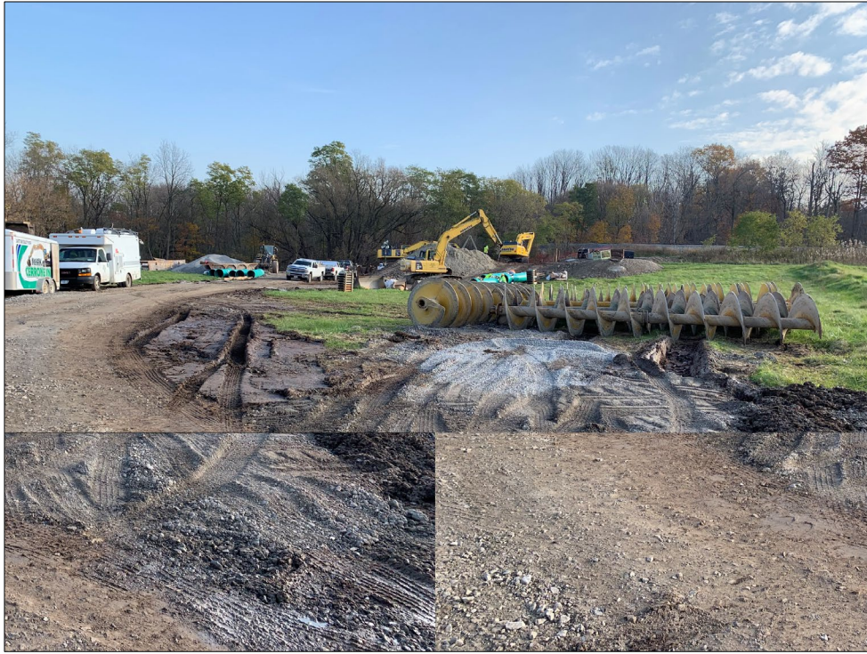
Photo 3 Construction/laydown area in northeast corner facing northeast
