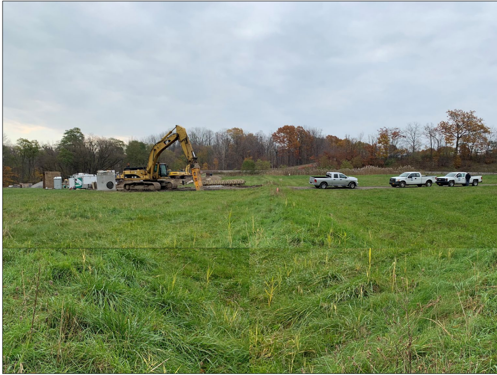
Photo 7 Site facing east along Drainage Swale B toward construction area
