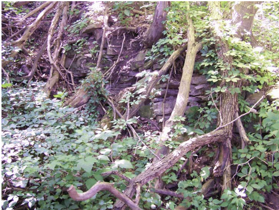
Figure 9-6. Photograph of the historic raceway wall west of the wall shown in Figure 9-5. View looking southwest. Photograph taken by Glenn May on July 14, 2008.
