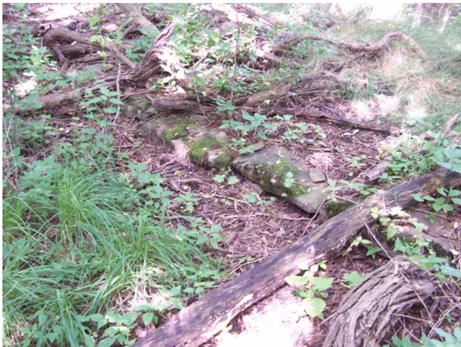
Figure 9-2. Photograph of the northern wall of the historic raceway on the eastern portion of the Dussault property. View looking northwest. Photograph taken by Glenn May on July 14, 2008.
