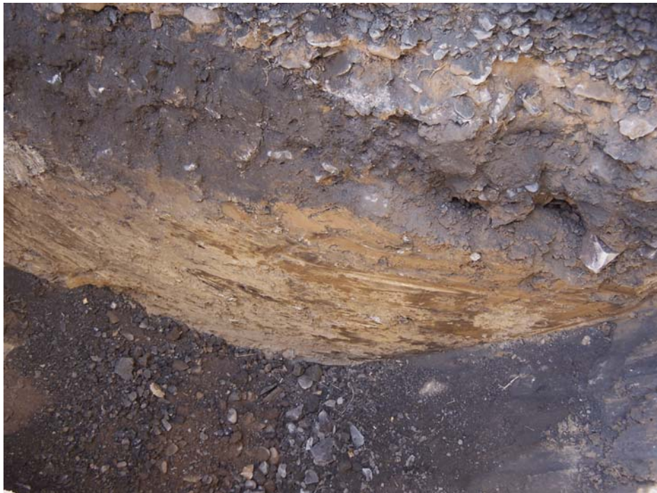
Figure 6-12. Photograph of the native silty clay (below the fill layer) in test pit SUB-80. Photograph taken by Glenn May on September 8, 2008.
