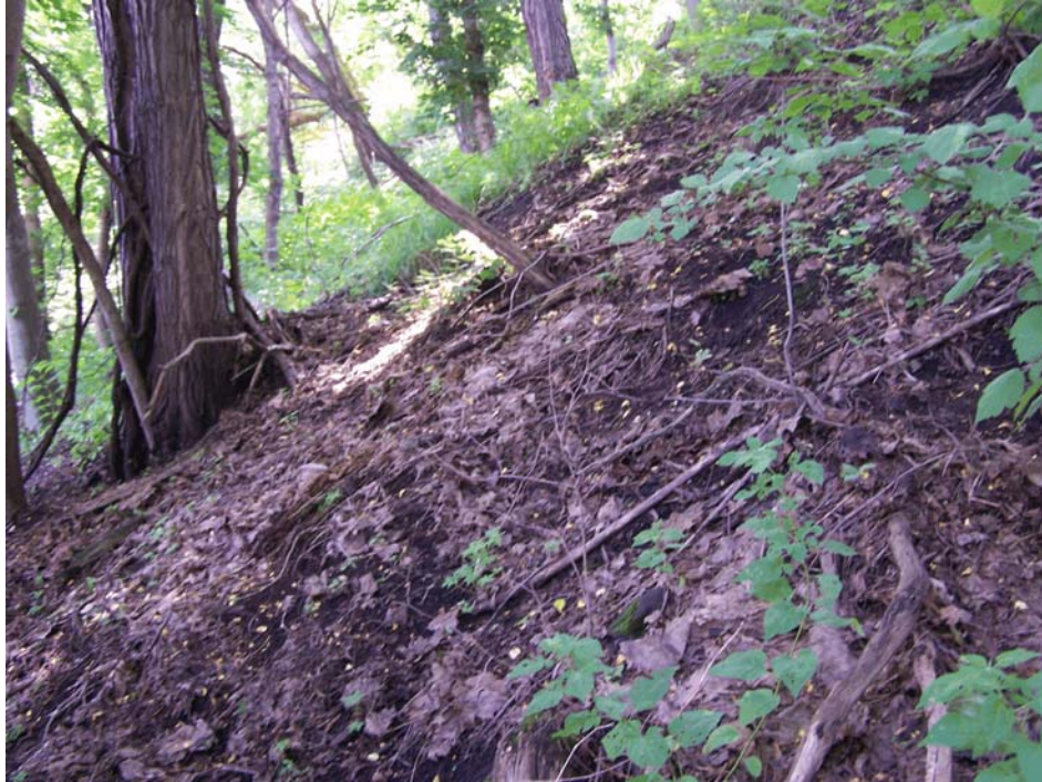
Figure 6-17. Photograph of the thick mantle of foundry sand overlying the Niagara Escarpment. View looking northeast. Photograph taken by Glenn May on July 14, 2008.
