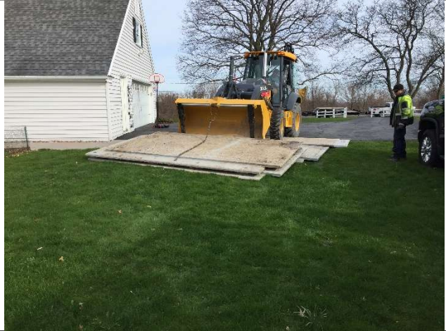
L3: Placing mats on property. View looking north.
