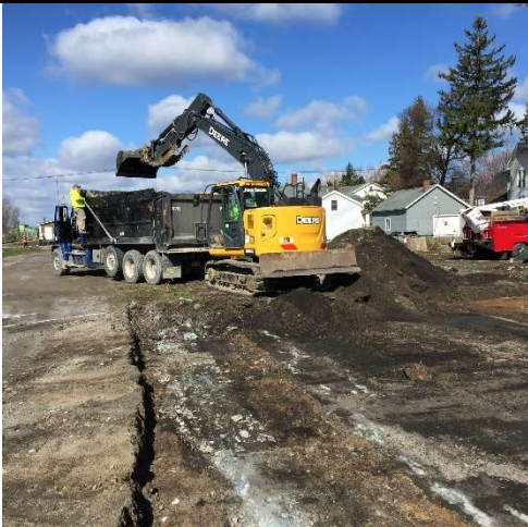
N15: Excavating 12" cut area. View looking west.
