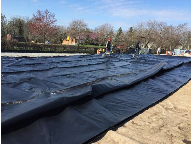
Staging Area: Installation of new liner to top of contaminated material pad. View looking southwest.
