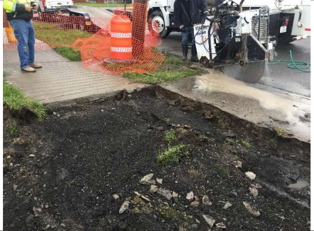
N15: Saw cutting concrete for removal. View looking northeast.
