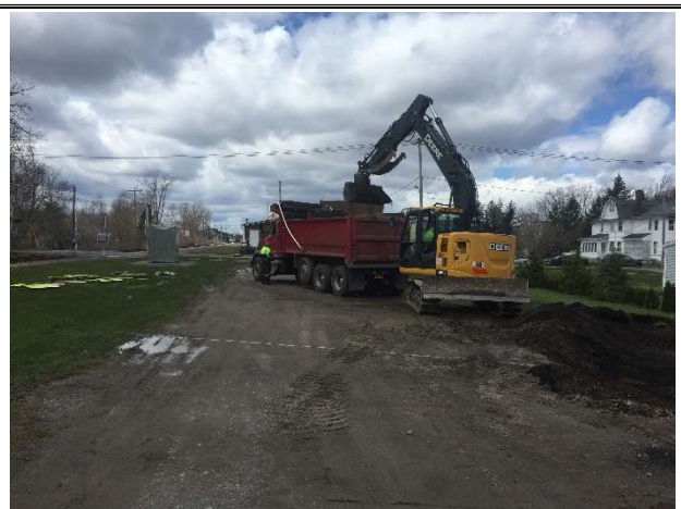
N15: Direct loading excavated material from the 18" cut area. View looking west.
