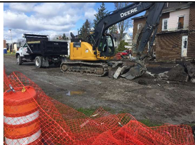
N15: Loading NVES truck with concrete for recycling. View looking northwest.
