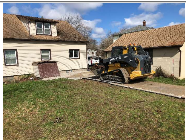
S6: Skid steer transporting excavated soil to trailer for transport to the staging area. View looking northwest.
