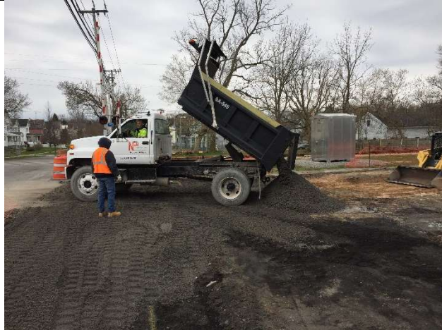
N15: NVES backfilling with stone at the east side of the property. View looking south.
