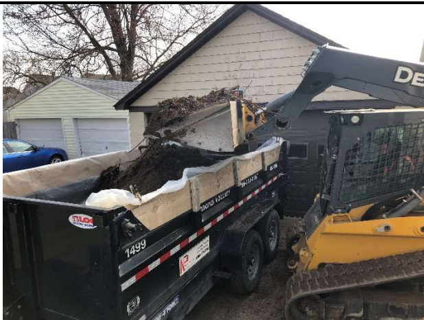
S6: NVES loading a trailer with excavated soil for transport to the staging area. View looking east.
