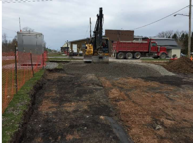
N15: NVES backfilling with stone at the west end of the property. View looking west.
