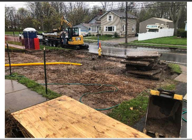
S6: Concrete sidewalk pulled for recycling. View looking southwest.
