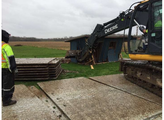
L3: NVES removing shed. View looking southeast.
