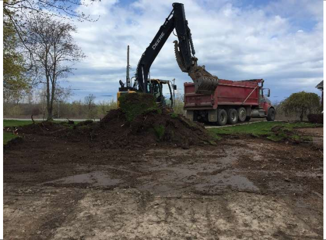
L3: NVES direct loading excavated material for disposal. View looking northeast.
