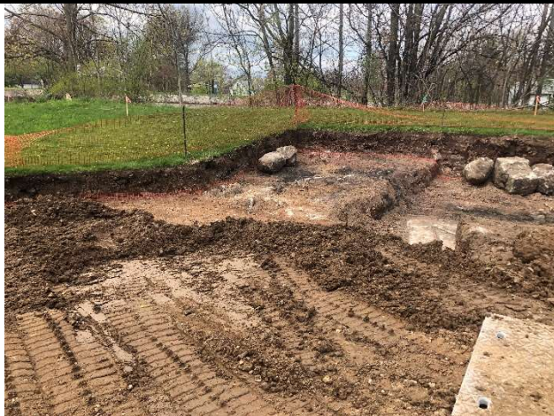
B1: NVES backfilling eastern excavation with common fill. View looking northwest.
