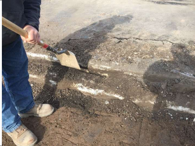
L3: NVES excavating along edge of driveway, which is asphalt over concrete. View looking west.
