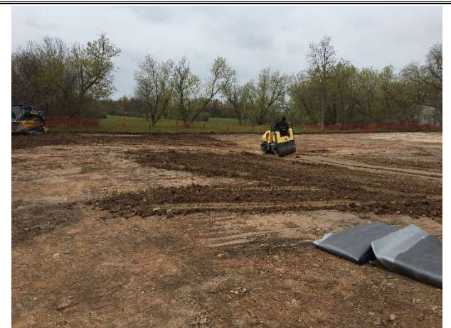
L3: NVES compacting common fill. View looking southwest.
