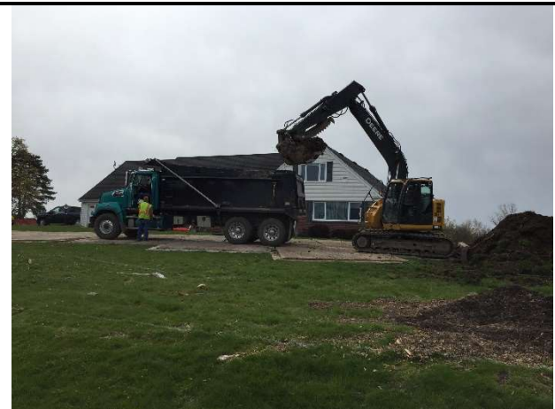
L3: NVES direct loading excavated material. View looking south.
