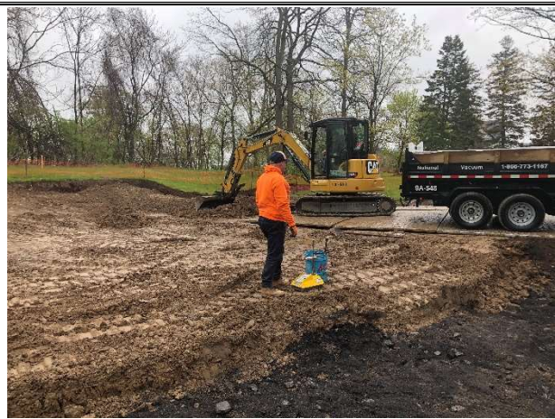
B1: NVES backfilling the northeast corner of the property, SJB performing compaction test. View looking east.
