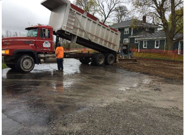
L3: NVES backfilling with common fill. View looking northeast.
