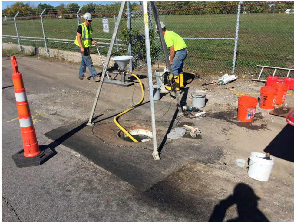
Photo 13 Stimm personnel injecting grout in manhole Walck MH-4 liner/structure voids.
