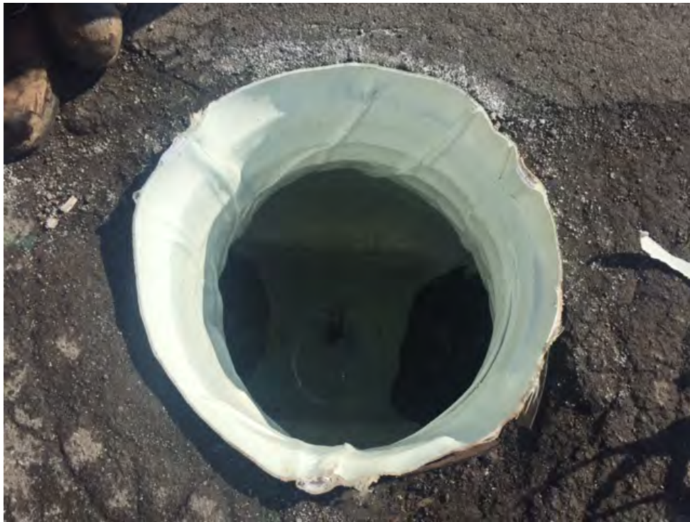
Photo 11 View of a completed manhole liner installation.
