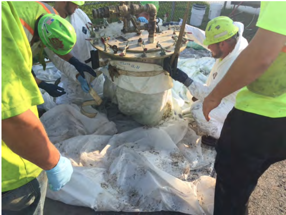
Photo 9 Arold personnel setting up to cure a manhole liner sock.
