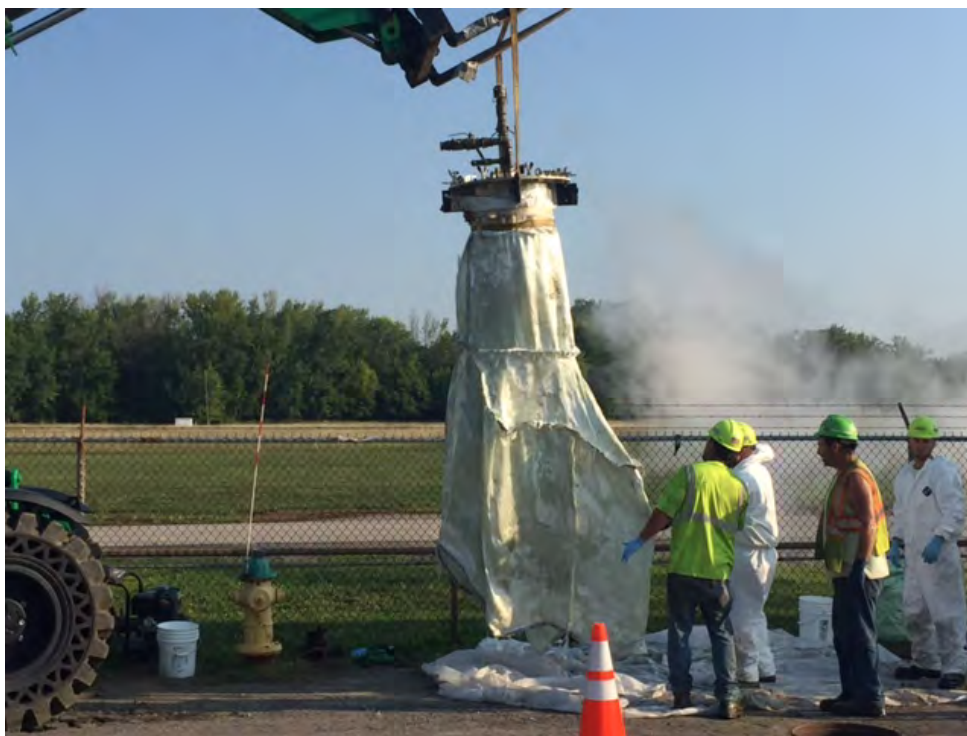
Photo 8 Arold personnel preparing to install a manhole liner sock at Walck MH-5.
