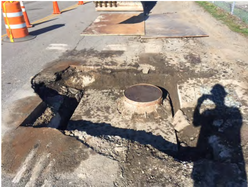
Photo 1 Manhole Walck MH-11 structure lid exposed.
