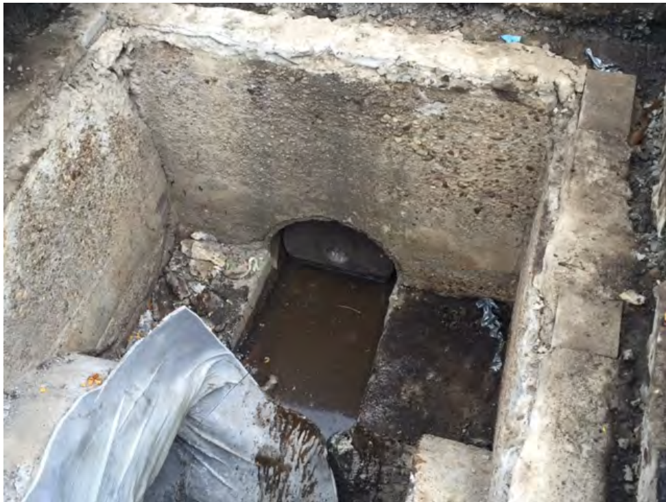
Photo 12 Manhole Walck MH-4 view north showing rubber sewer plug.
