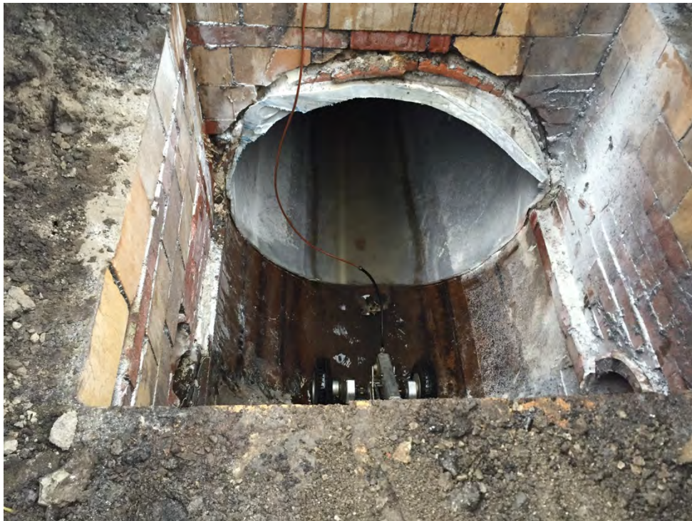
Photo 6 CIPP liner trimmed in manhole Walck MH-11.
