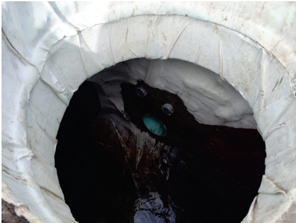
Photo 15 Durez NT discharge pipe and bulkhead.
