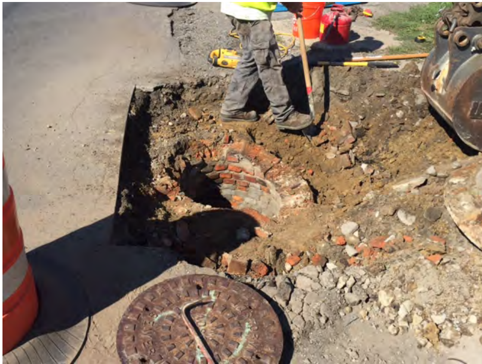
Photo 3 Opening of manhole Walck MH-2 structure.
