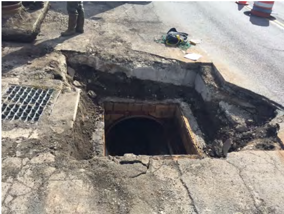
Photo 2 Manhole Walck MH-11 structure lid removed.
