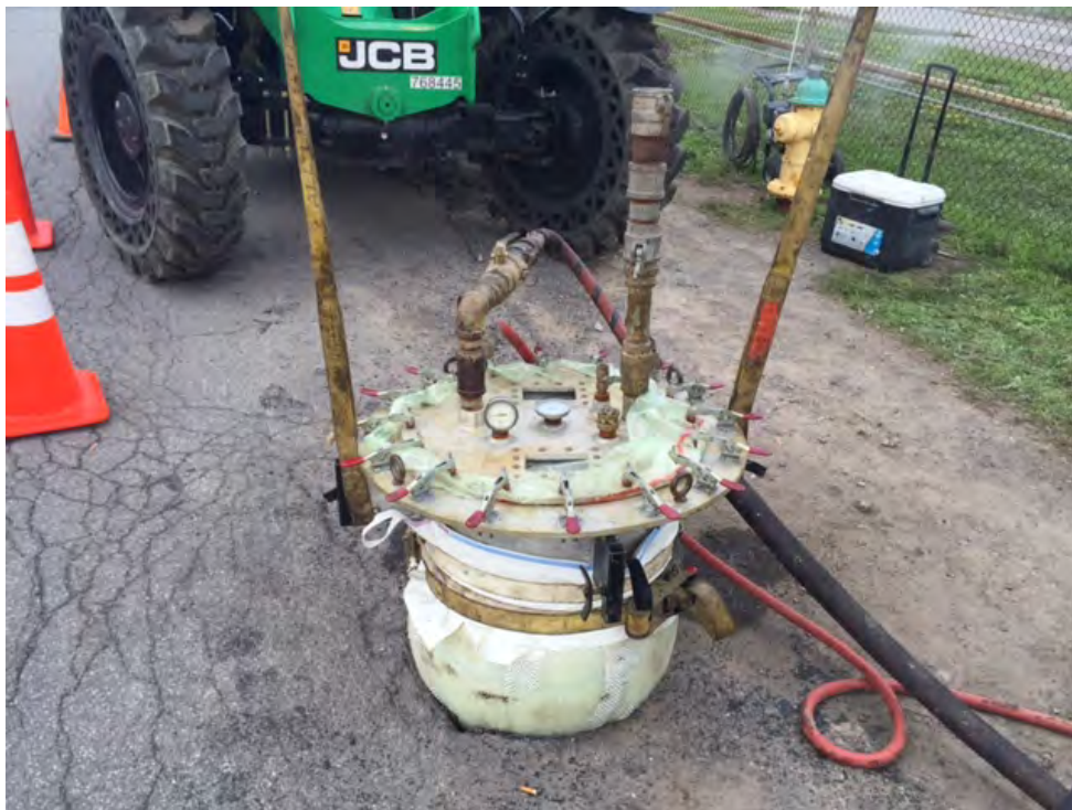
Photo 10 A manhole liner sock steam curing.
