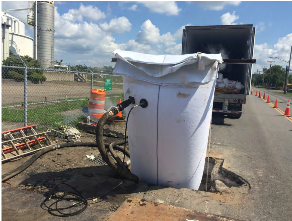
Photo 5 CIPP liner curing in manhole Walck MH-11.
