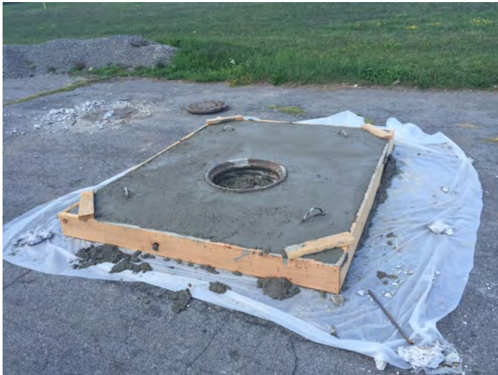
Photo 4 Manhole Walck MH-4 new structure lid.
