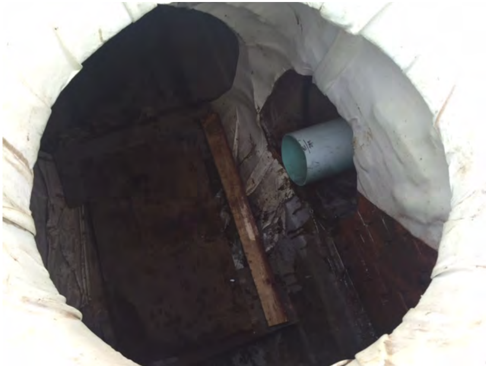
Photo 14 Durez NT discharge pipe extended into the WRS System.
