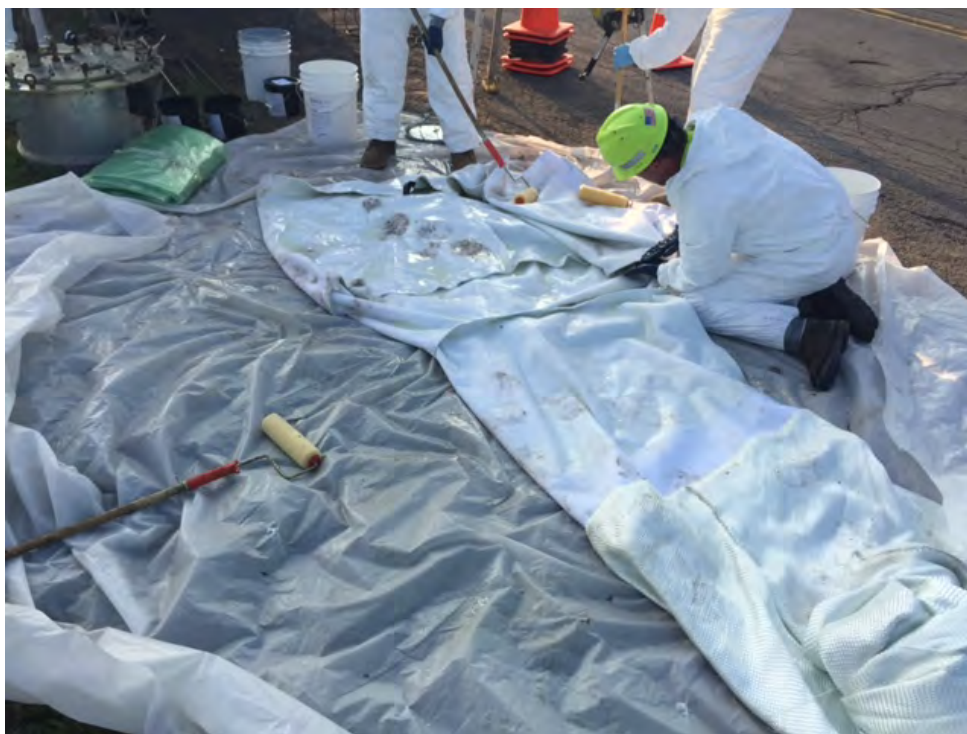
Photo 7 Arold personnel applying resin to manhole liner sock.
