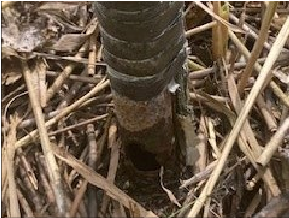
Photo 3 View of P-16 with hole in riser observed on July 1, 2021.
