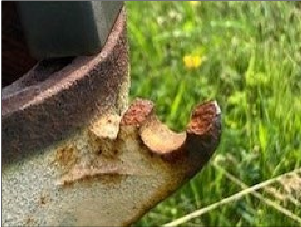
Photo 1 View of NP-8 observed on July 7, 2021 with broken hasp.
