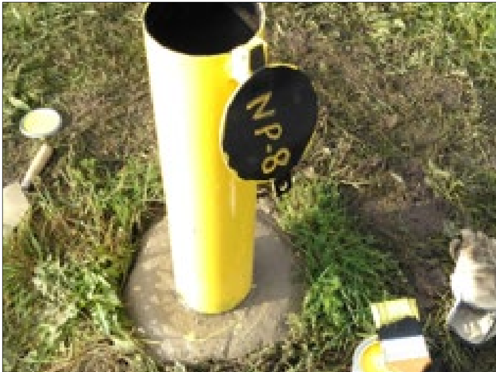
Photo 2 View of NP-8 with new locking 6-inch protective casing and concrete pad installed on October 6, 2021.
