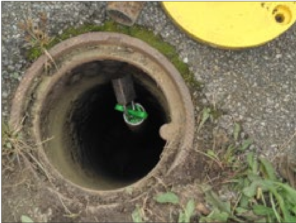
Photo 5 View of T-11B following removal of the top ~3 inches of corroded riser on October 6, 2021.
