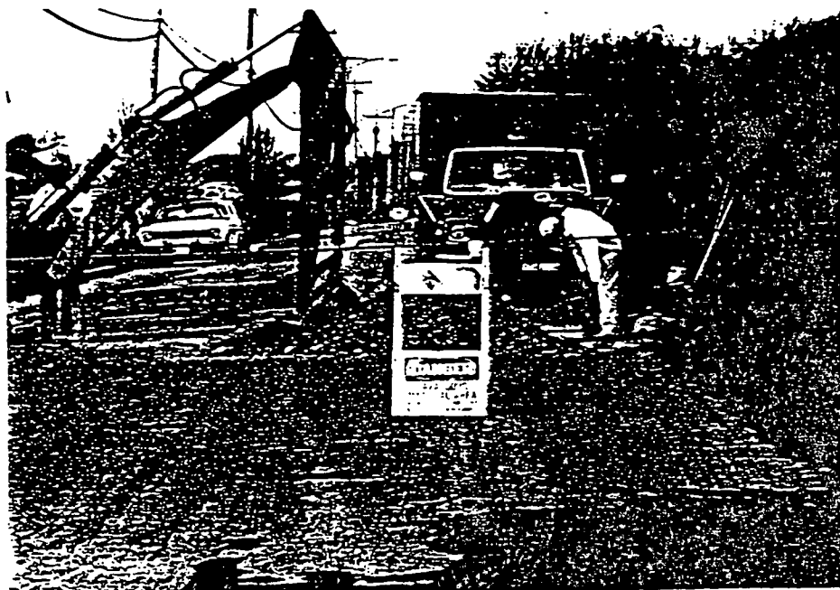
Storm Sewer Work on Frontier Avenue.
