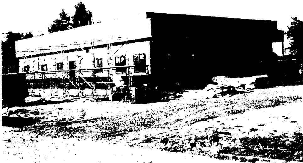
Fig. 4 Work on the Love Canal Administration Building is expected to be complete in November 1986. This building will serve as a support building for the Leachate Treatment Plant DEC Staff.
