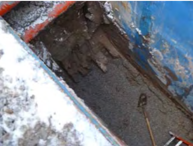
Photo 9: Feb. 03, 2011: Clay and stone bedding above sanitary sewer pipe approx. 15 feet east of manhole at 96 th Street.
