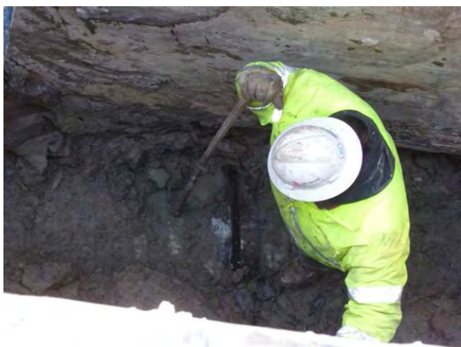
Photo 29: Feb. 09, 2011: Preparing to remove next 5-foot section of concrete pipe.
