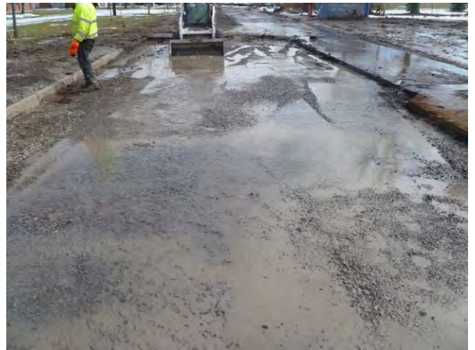
Photo 46: Feb. 18, 2011: Area compacted and ready to receive temporary asphalt patch.
