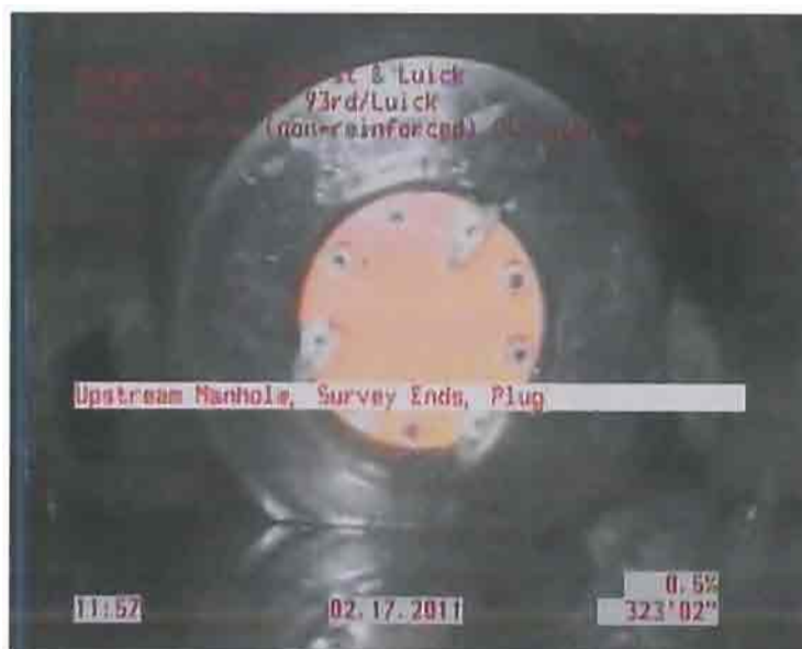
Photo: 5_1_2_18022011_105909_A.JPG, VCR No.: X 323.2FT, Upstream Manhole, Survey Ends / Plug
