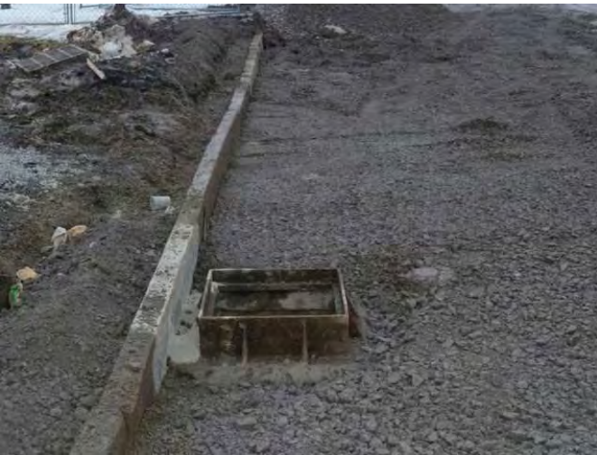
Photo 45: Feb. 17, 2011: Catch basin installed, roadway curbing installed, sub-base installed.
