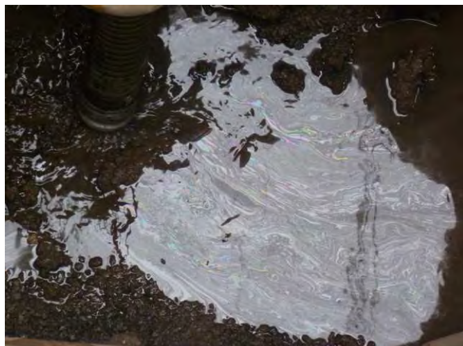
Photo 14: Feb. 04, 2011: Vacuuming excavation water with sheen.
