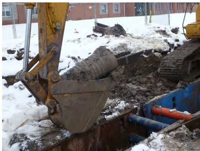
Photo 22: Feb. 07, 2011: Removing next 5-foot section of concrete sanitary sewer piping.
