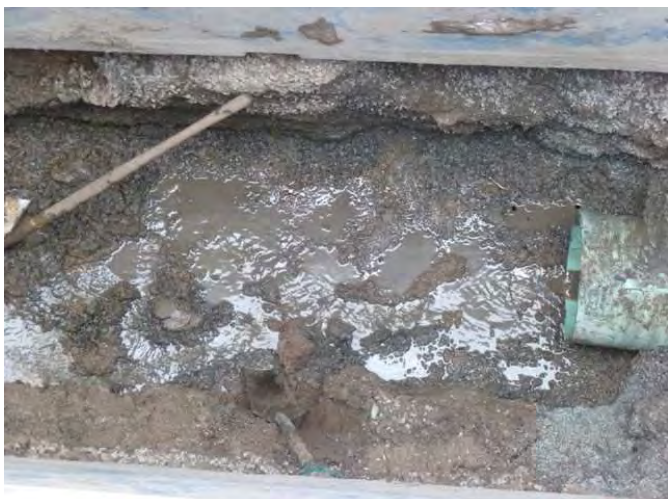
Photo 13: Feb. 04, 2011: Excavation nearly dewatered. Note black dots near pipe end that appears to be a NAPL-like material. Approx. 10 ft west of manhole at 96 th Street.
