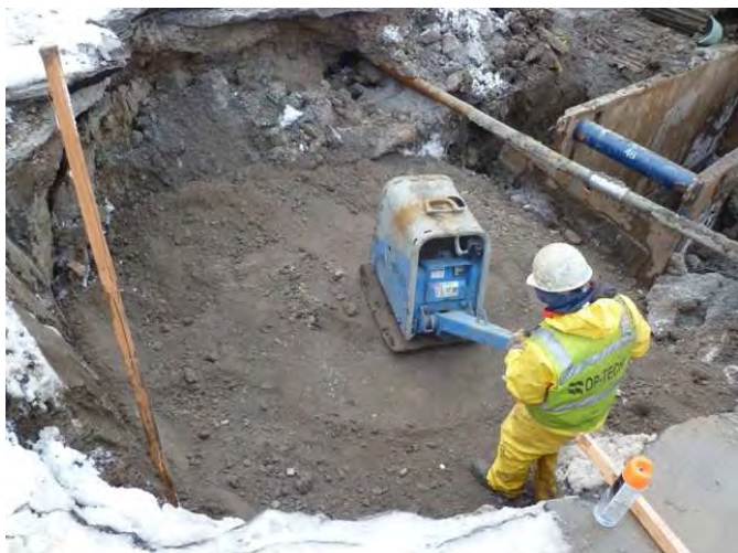
Photo 19: Feb. 05, 2011: Backfilling of 1 st 14-foot section of new pipe continues.
