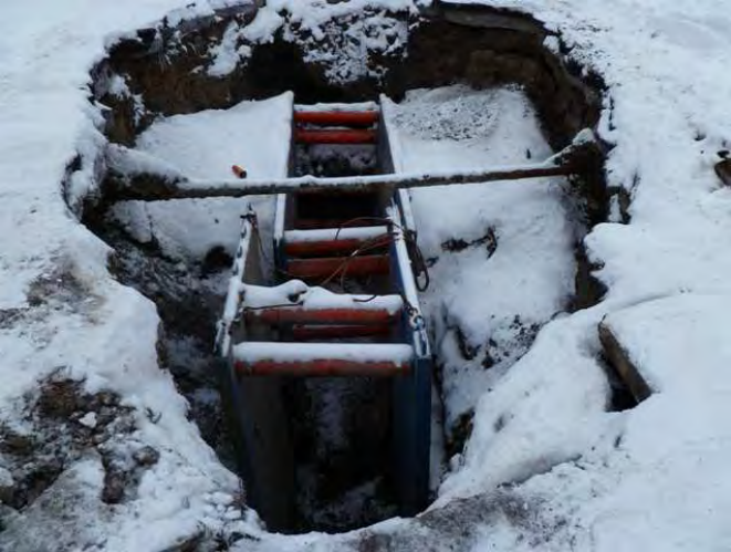
Photo 1: Feb. 01, 2011: Excavation at start of work activities
