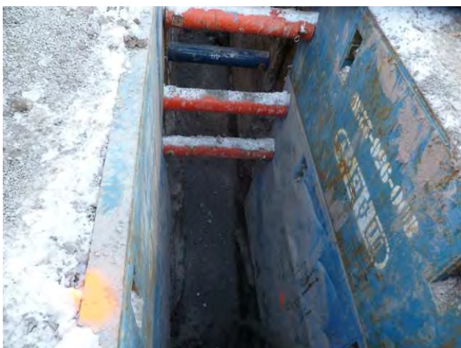
Photo 17: Feb. 04, 2011: Two feet of new bedding installed.
