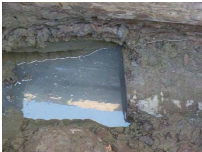
Photo 32: Feb. 09, 2011: Bedding location of 5-foot section removed in Photo's 29, 30 and 31.
