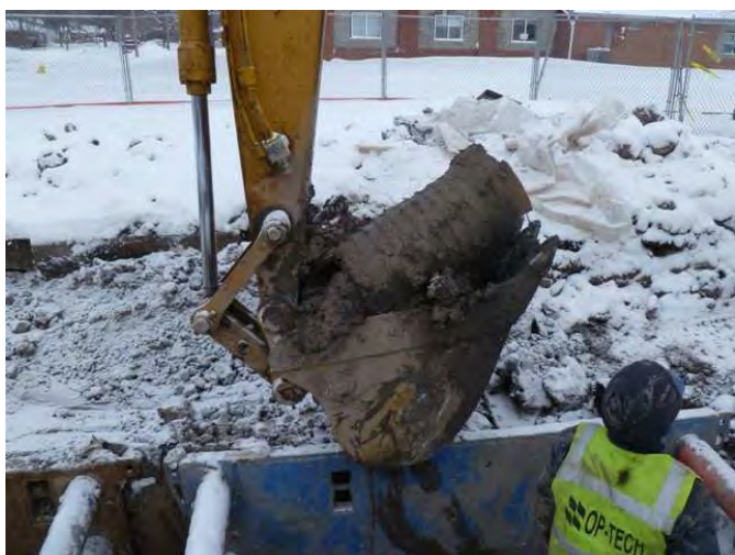
Photo 23: Feb. 08, 2011: Removing another 5-foot section of pipe.
