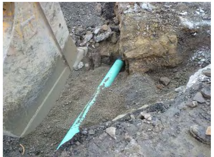
Photo 42: Feb 16, 2011: Repaired storm sewer line.
