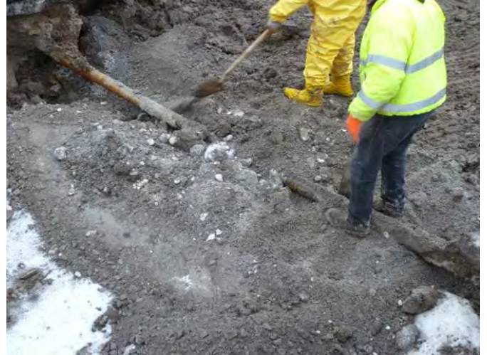
Photo 38: Feb. 14, 2011: Hand backfilling around gas line.
