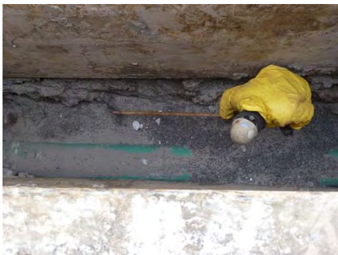
Photo 27: Feb. 08, 2011: Backfilling 2 nd 14-foot section.
