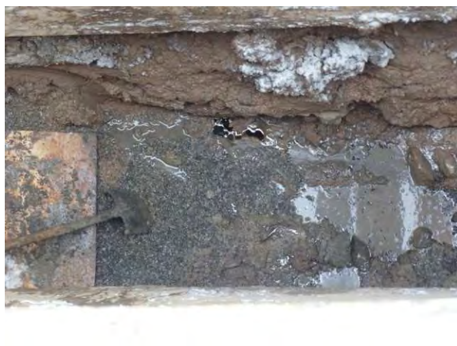
Photo 24: Feb. 08, 2011: Under-bedding and clay removed to extent possible. Note NAPL-like material.
