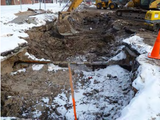
Photo 37; Feb. 11, 2011: Backfilling activities continue.
