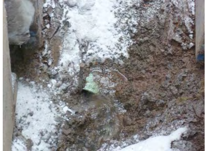
Photo 2: Feb. 01, 2011: Temporary pipe placed by City contractor with sanitary flow.
