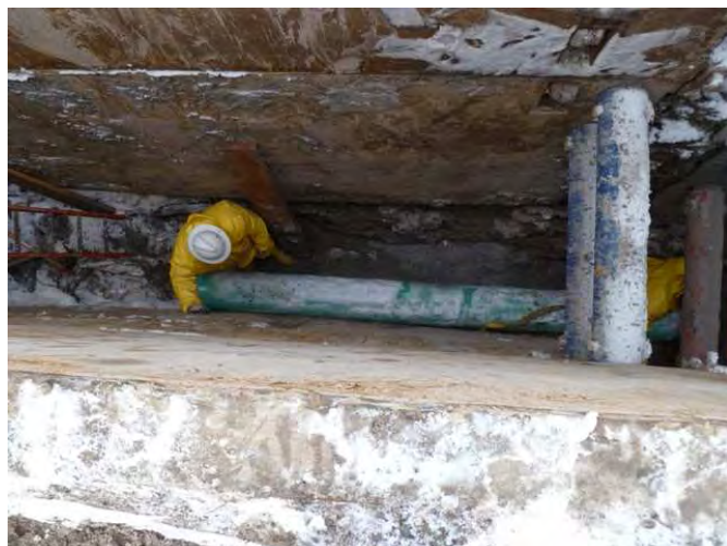
Photo 26: Feb. 08, 2011: Installing 2 nd 14-foot section of new PVC pipe.
