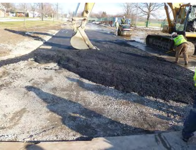
Photo 47: Feb. 18, 2011: Installing temporary asphalt patch.
