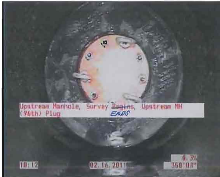
Photo: 1_1_2_17022011_091413_A.JPG, VCR No.: X 349.5FT, Upstream Manhole, Survey Begins / Upstream MH (96th) Plug
