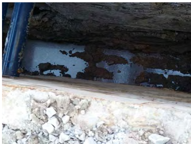
Photo 16: Feb. 04, 2011: Under pipe bedding and clay removed to the extent possible. Approx. 2 ft of material removed below pipe.
