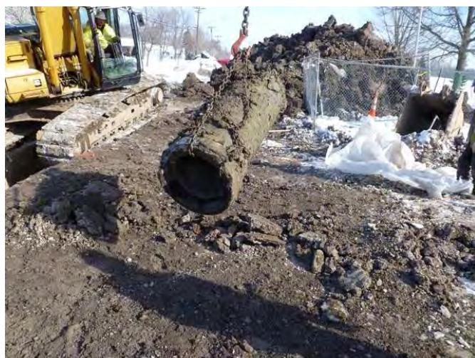
Photo 30: Feb. 09, 2011: Removing next 5-foot section with in-pipe sediments still in pipe.
