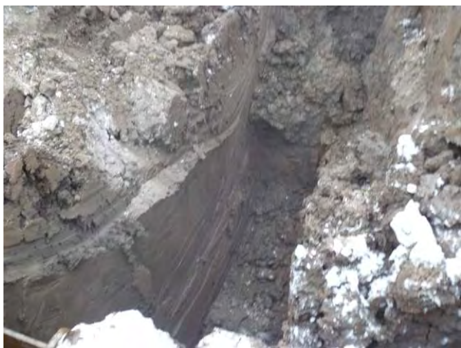
Photo 21: Feb. 07, 2011: Continuing to excavate; clay soil above pipe.
