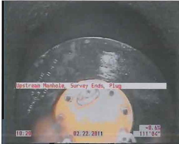
Photo: 6_1_2_23022011_092256_A.JPG, VCR No.: X 111.35FT, Upstream Manhole, Survey Ends / Plug
