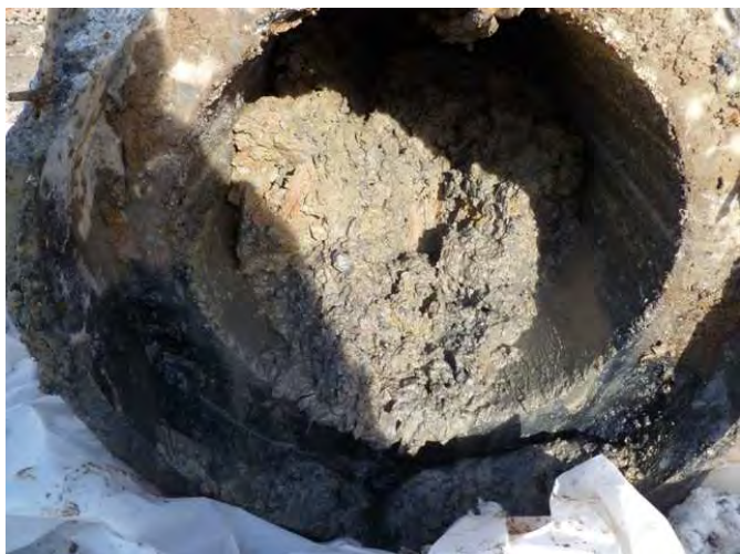
Photo 31: Feb. 09, 2011: Sediments inside of concrete sanitary sewer pipe.
