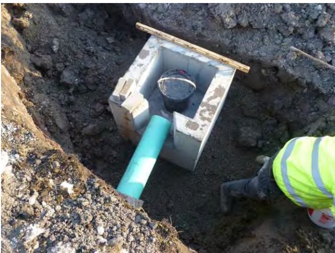
Photo 41: Feb. 15, 2011: New storm catch basin installed.
