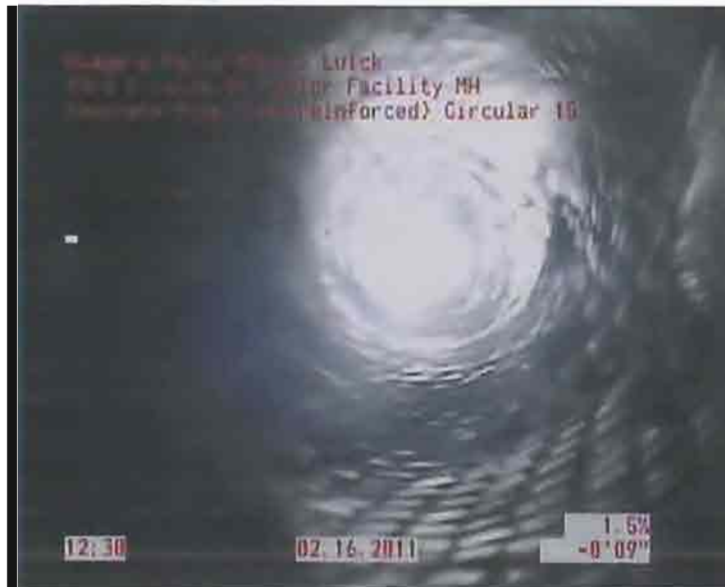
Photo: 3_1_1_17022011_113243_A.JPG, VCR No.: X 0FT, Reversal Inspection / Inspection towards Senior Facility MH from 93rd & Luick ave.
