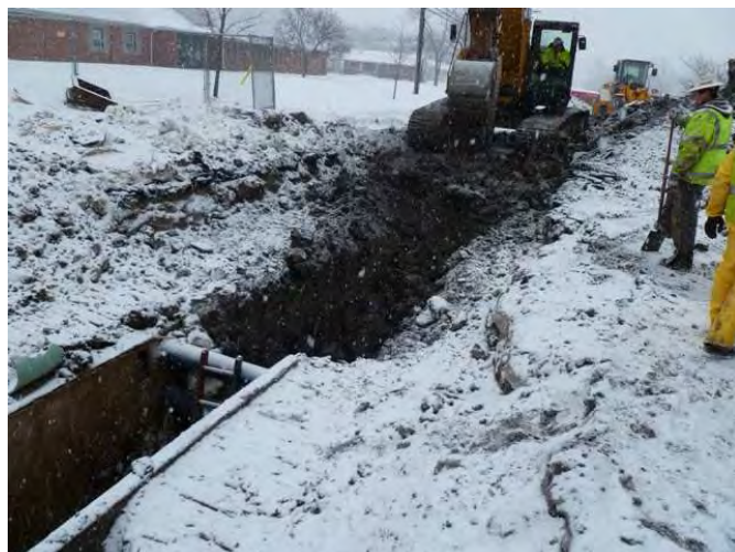
Photo 20: Feb. 05, 2011: Excavating to place trench boxes for next section of pipe.
