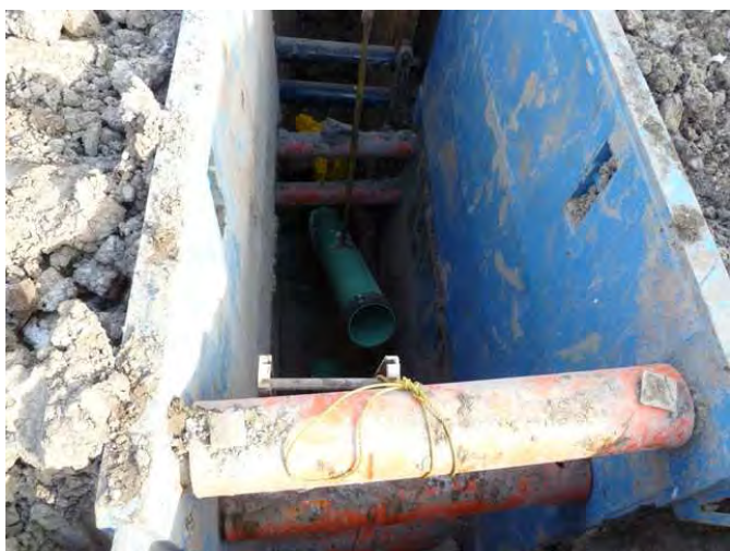
Photo 35: Feb. 10, 2011: Placing last section of new PVC pipe.
