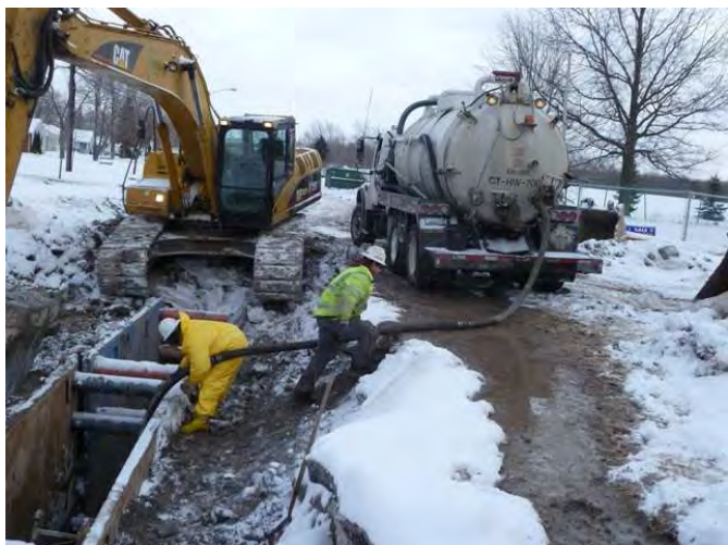
Photo 25: Feb 08, 2011: Vacuuming water and NAPL-like material from excavation.
