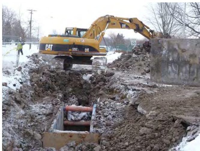
Photo 28: Feb. 09, 2011: Excavating to place trench box for next section of piping.
