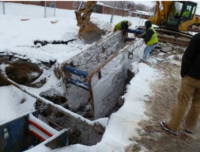
Photo 3: Feb. 02, 2011: Placing safety trench box. Note 4-inch gas line transecting excavation.
