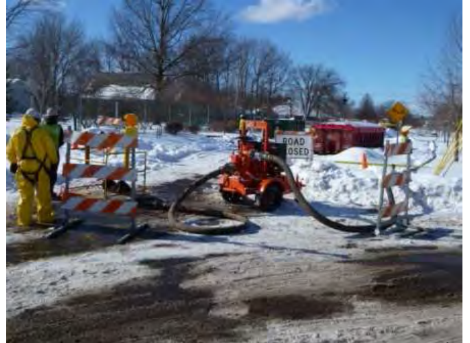
Photo 8: Feb. 03, 2011: Bypass activities from manhole at 97 th Street and Colvin Blvd going west to manhole at 96 th Street and Colvin Blvd.
