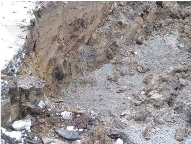
Photo 39: Feb. 14, 2011: Area for repair of street catch basin; note storm sewer pipe in excavation sidewall.
