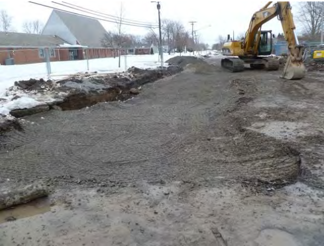
Photo 43: Feb. 16, 2011: Roadway sub-bas being installed and compacted.
