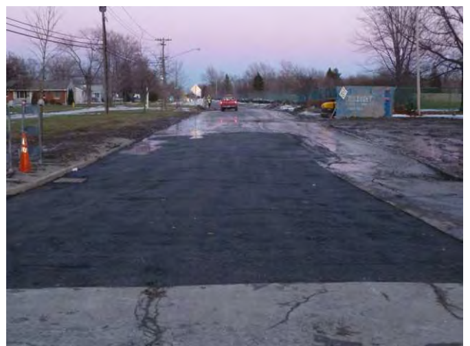
Photo 48: Feb. 18, 2011: Asphalt patch installed; road being opened to traffic.
