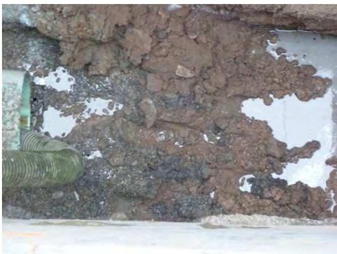
Photo 15: Feb. 04, 2011: Under pipe bedding and clay removed to the extent possible.
