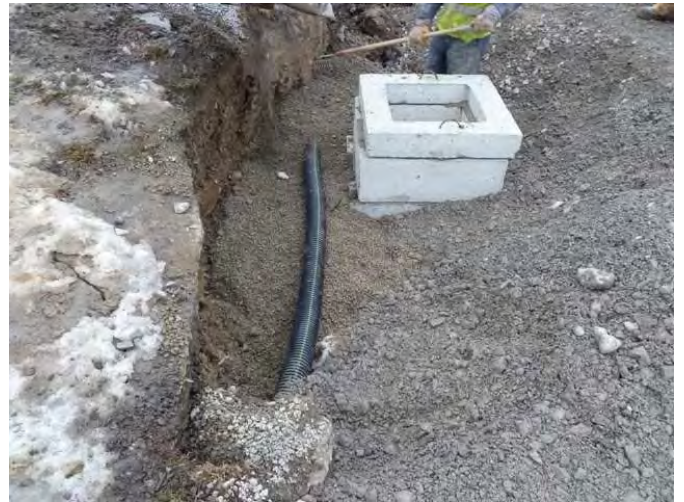
Photo 44: Feb. 16, 2011: Storm catch basin raised to grade and roadway french drain installed.
