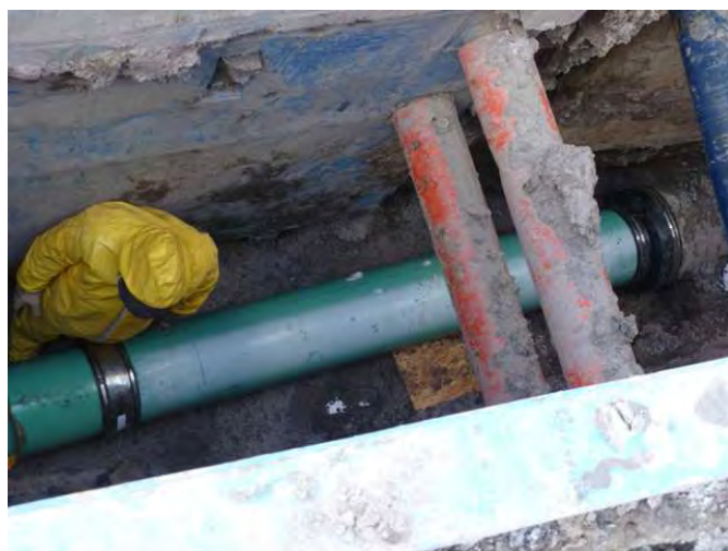
Photo 36: Feb. 10, 2011: Last section of new pipe connected to existing concrete pipe.
