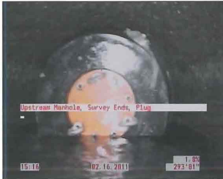
Photo: 4_1_4_17022011_141815_A.JPG, VCR No.: X 293.1FT, Upstream Manhole, Survey Ends / Plug
