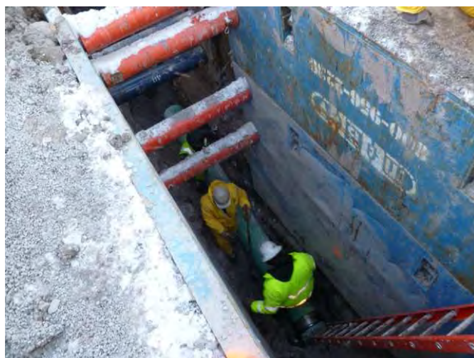
Photo 18: Feb 04, 2011: First 14-ft section of new pipe installed.
