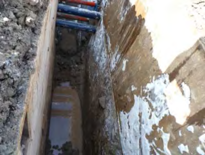
Photo 7: Feb. 03, 2011: Excavation conditions above sanitary sewer pipe; note clay materials.
