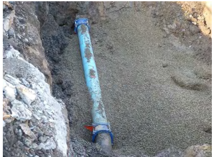
Photo 40: Feb. 15, 2011: Repaired 8-inch water line.
