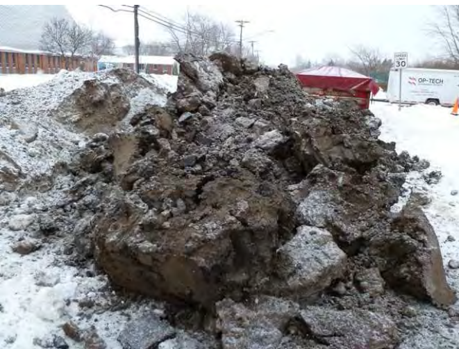
Photo 5: Feb. 02, 2011: Clay soil excavated from above sanitary sewer pipe.
