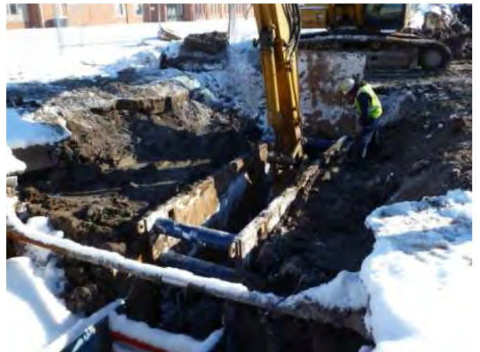
Photo 6: Feb. 03, 2011: Continuing to excavate and secure trench box.
