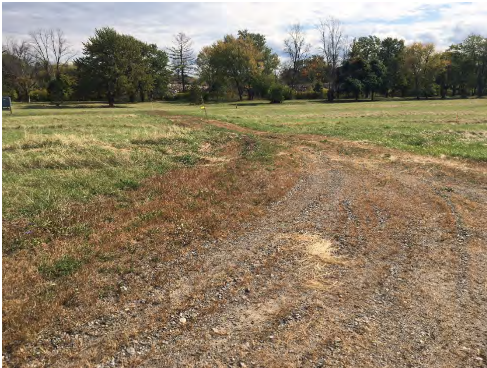
Photo 4 - View east of depression in access road before regrading
