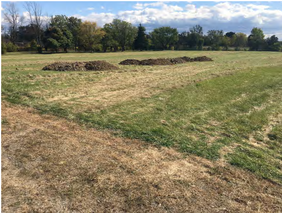
Photo 5 - View southeast of topsoil brought in to regrade cap
