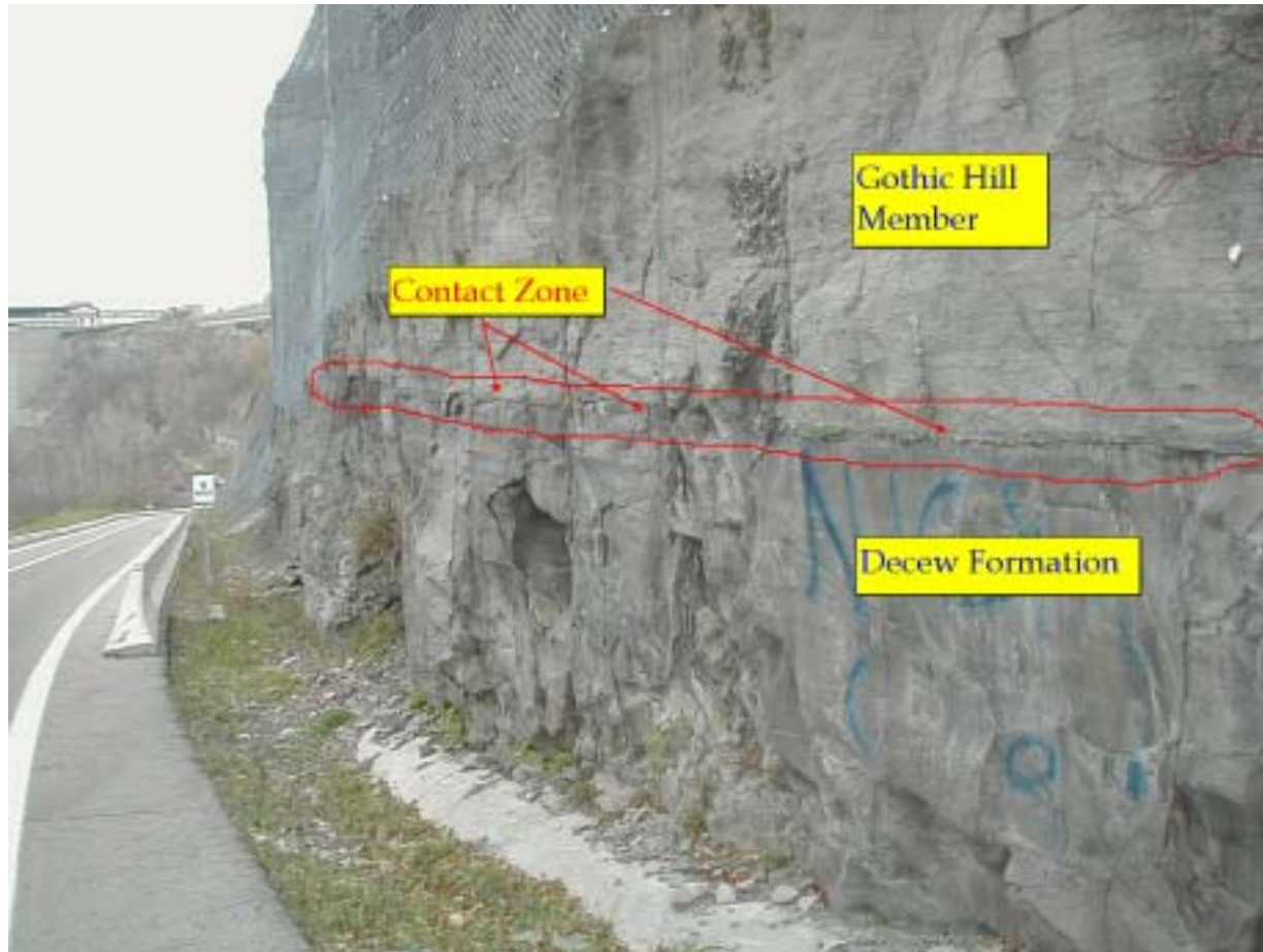
Photograph 10. Contact between Gothic Hill Member of the Gasport Formation and the DeCew Formation. Note the massive nature of each unit and overall lack of bedding plane fractures. NYPA Access Road.
