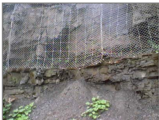
Photo 11, left. GF-S14, at the Irondequoit / Renaldi contact. Renaldi is the more fractured formation. This seep is about 30 feet wide. "Same as last year."
