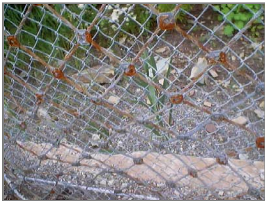
Photo 15, left. Rust on fencing at GF-S4 and Culvert 3 is caused by road salt in plow-thrown snow.
