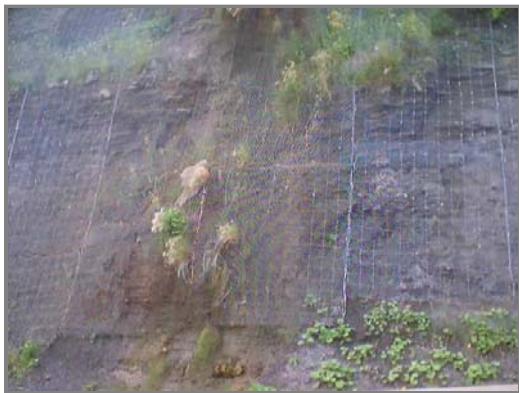
Photo 9, left. GF-S2, moist rock wall, vegetation growing on the fencing, except for 1-3 gpm flow, it's "the same as last year."
