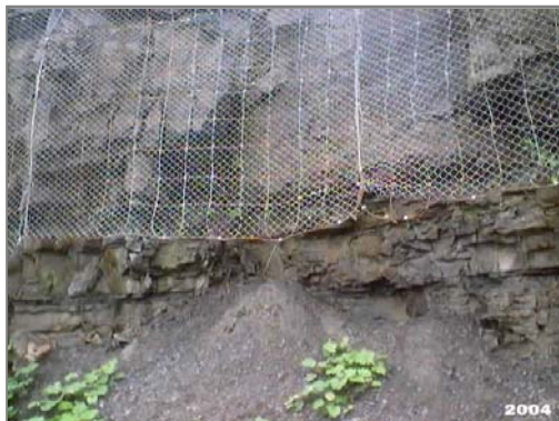
NYSDEC 2004: GF-S14, at the Irondequoit / Renaldi contact. Renaldi is the more fractured formation. This seep is about 30 feet wide. "Same as last year."
