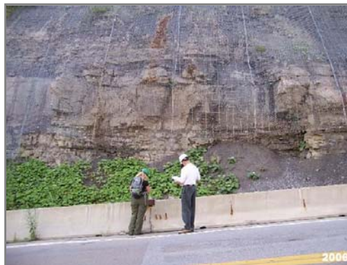
CRA 2004: Seep 14. Approximately 80' to 100' south of the south fence line of seep 3. Wet face on Reynales approximately 30' wide. Slight dripping originates from the Irondequoit/Reynales contact. No action required. Same conditions as 2000-2003.
