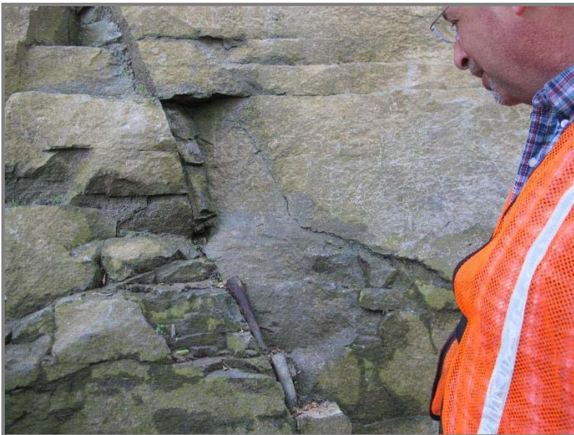
9:08 AM. Matt Forcucci pointed out two pieces of pipe. A galvanized pipe runs under the right hand edge, collecting water.
