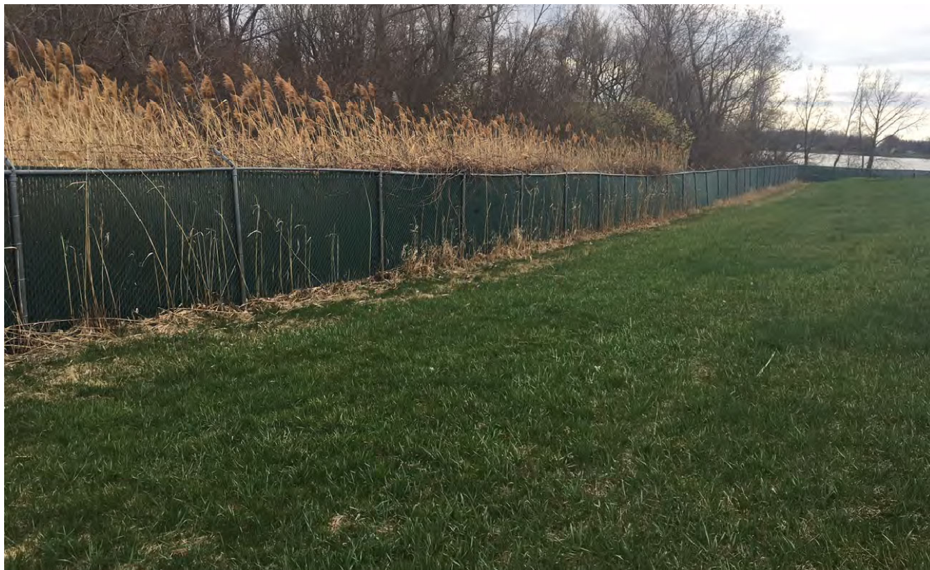
Figure 15: View of the landfill's eastern fence.
