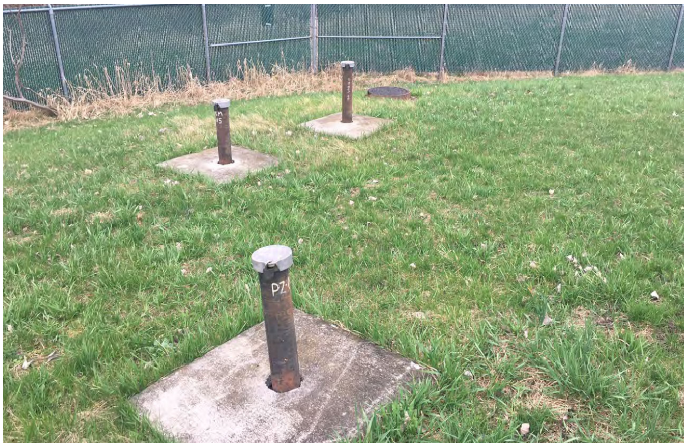
Figure 23: A cluster of monitoring wells on the eastern edge of the landfill.
