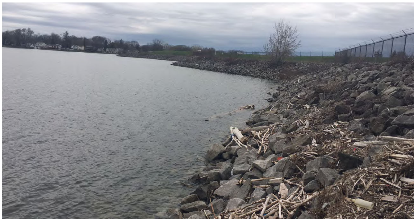
Figure 16: Embankment on the southern edge of the landfill.
