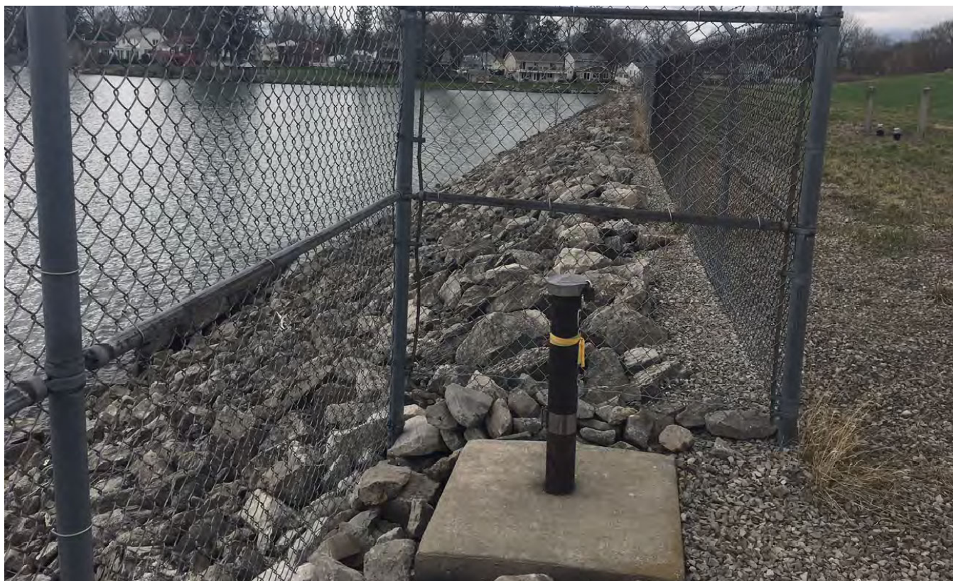
Figure 21: Closeup of a monitoring well on the landfill's southern edge.
