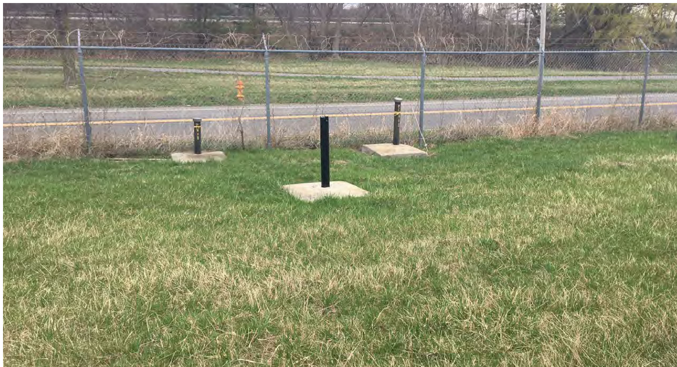
Figure 22: A cluster of monitoring wells on the landfill's northern edge.
