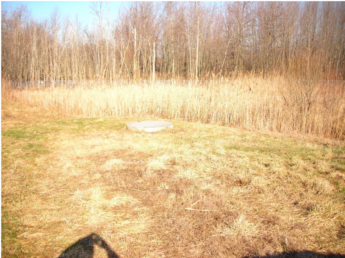
Photo 2: Taken from north side of landfill facing northwest near wet well D.
