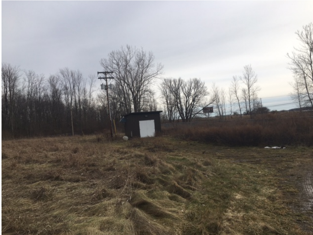
View of landfill control building, facing southeast.
