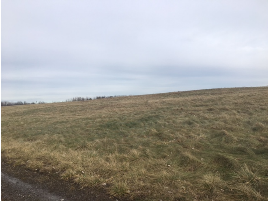
View of west side of the landfill cap, facing north.
