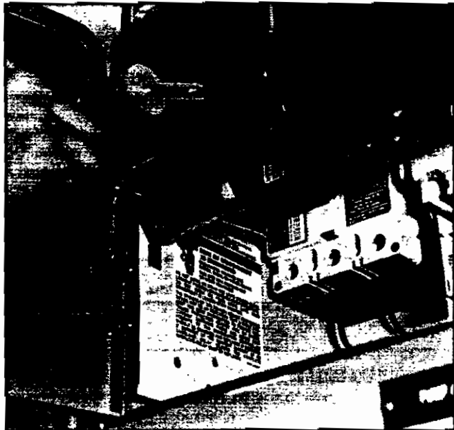
Fig. 25 HMCP Magnetic Adjustment
