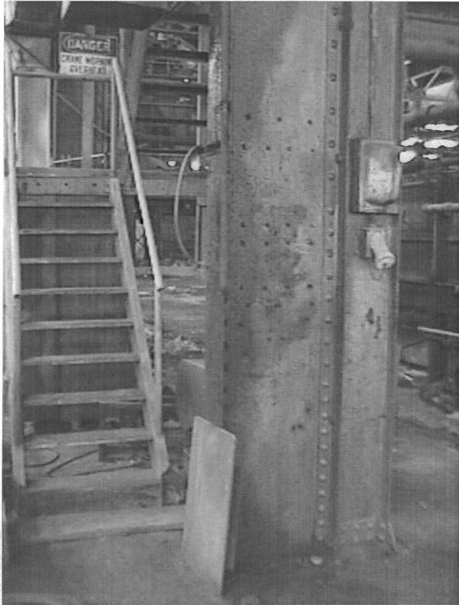
Photograph 21 - Building 4 & 9 - Typical Built-up Column
