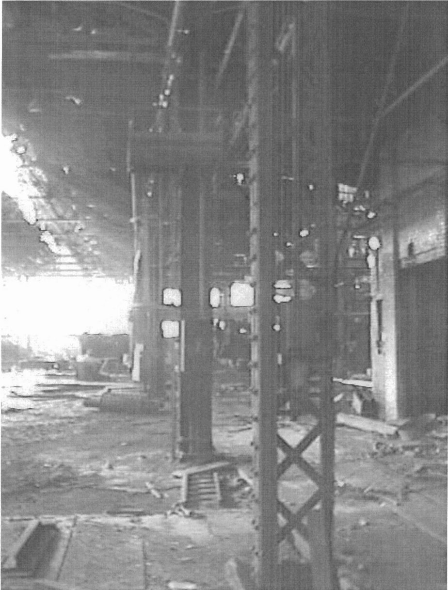
Photograph 15 - Buildings 6 & 8 - Typical Built-up Columns along Building 3 interface - facing south - Note furnace in background
