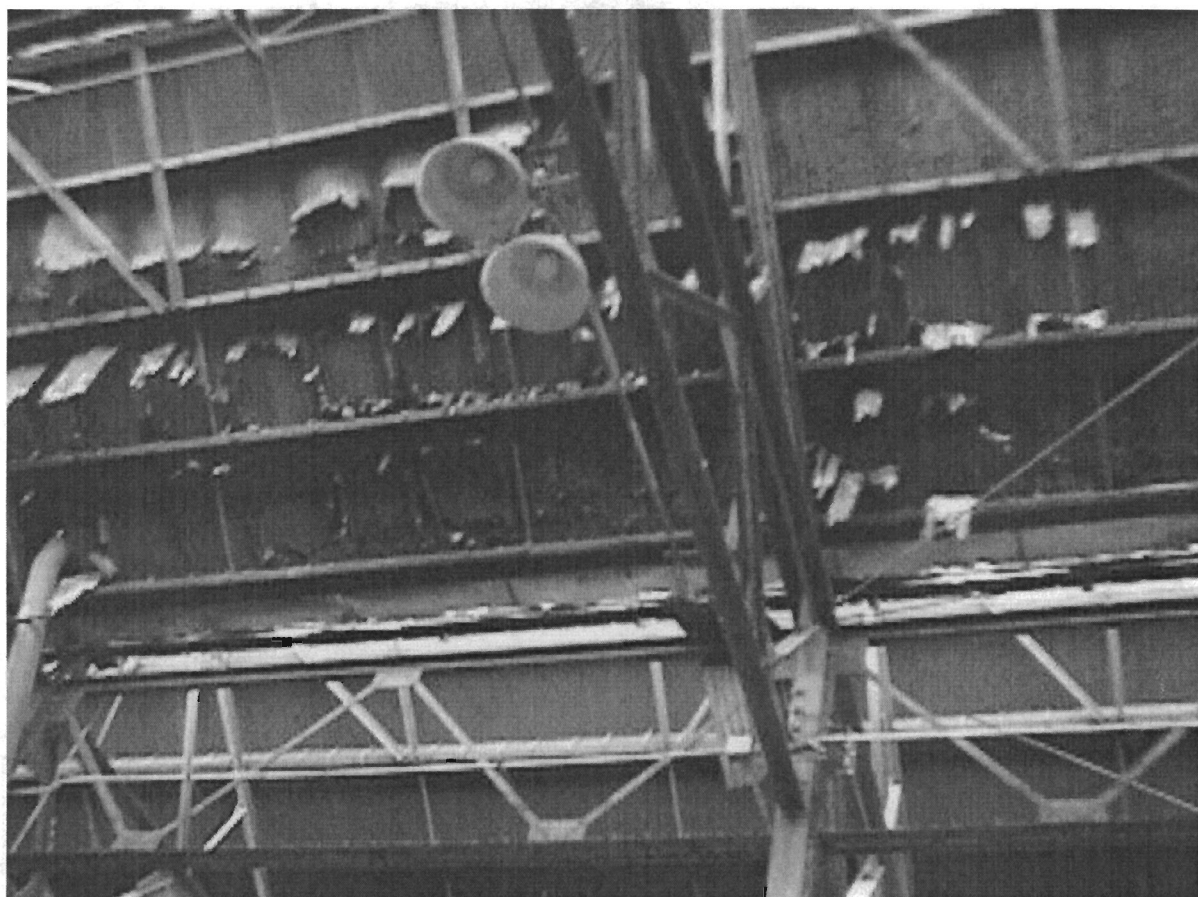
Photograph 19 - Buildings 4 & 9 - Typical peeling of roof material
