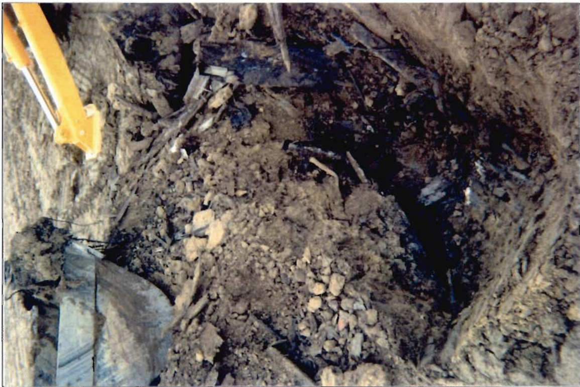
D-6 Holiday Park – Area 3. Test pit C in golf course expansion area (additional investigation). August 25, 1998.
