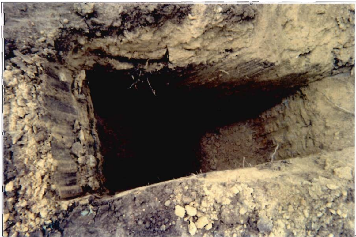
D-8 Holiday Park – Area 3. Test pit F in golf course expansion area (additional investigation). August 25, 1998.
