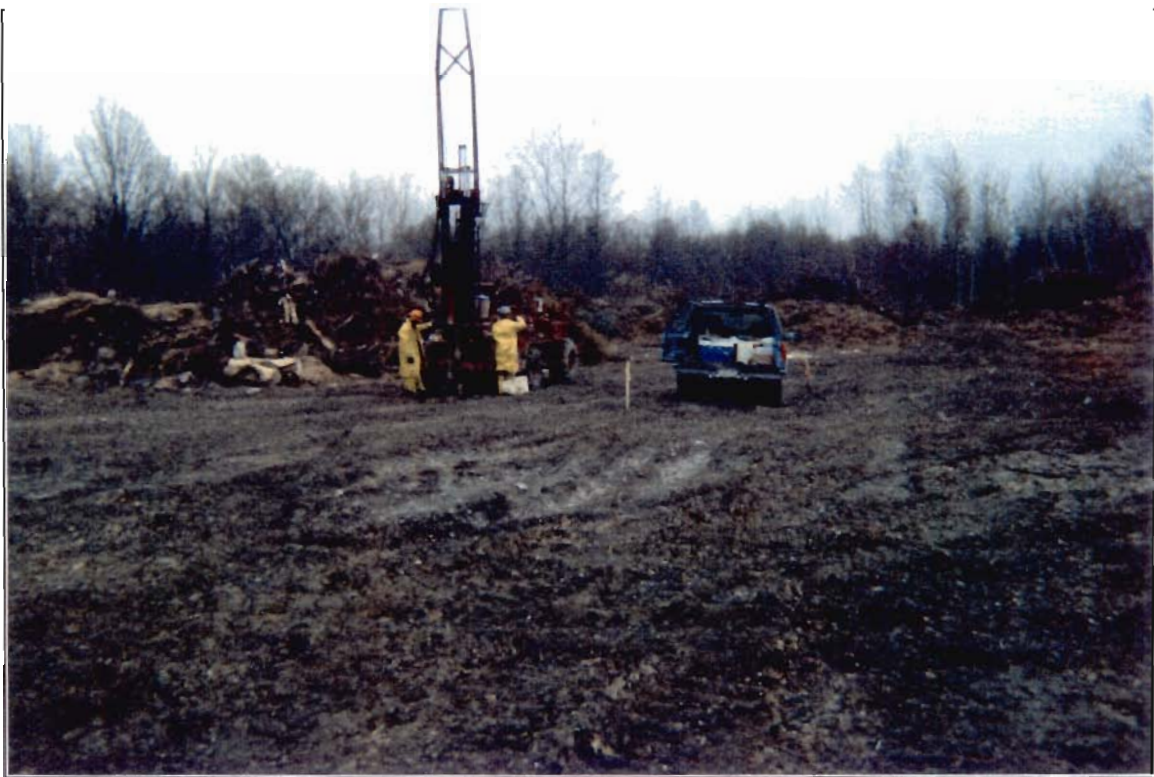
D-1 Holiday Park – Area 2. Facing southeast. Drilling rig at boring location HP2-B1. Location within recycling area. April 8, 1998.
