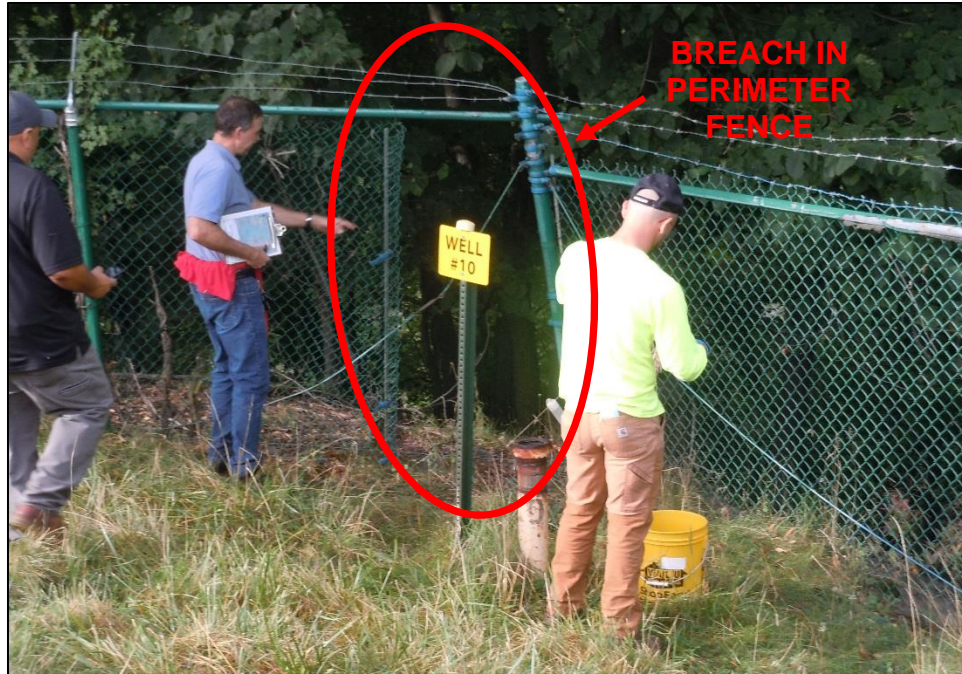
Breach in southern landfill perimeter fenceline near well VDM-10.
