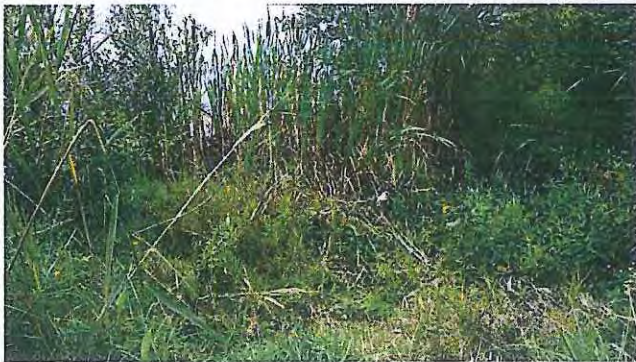
Overflow Weir (Dry)
