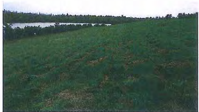
Lakeside Slope of Capped Area
