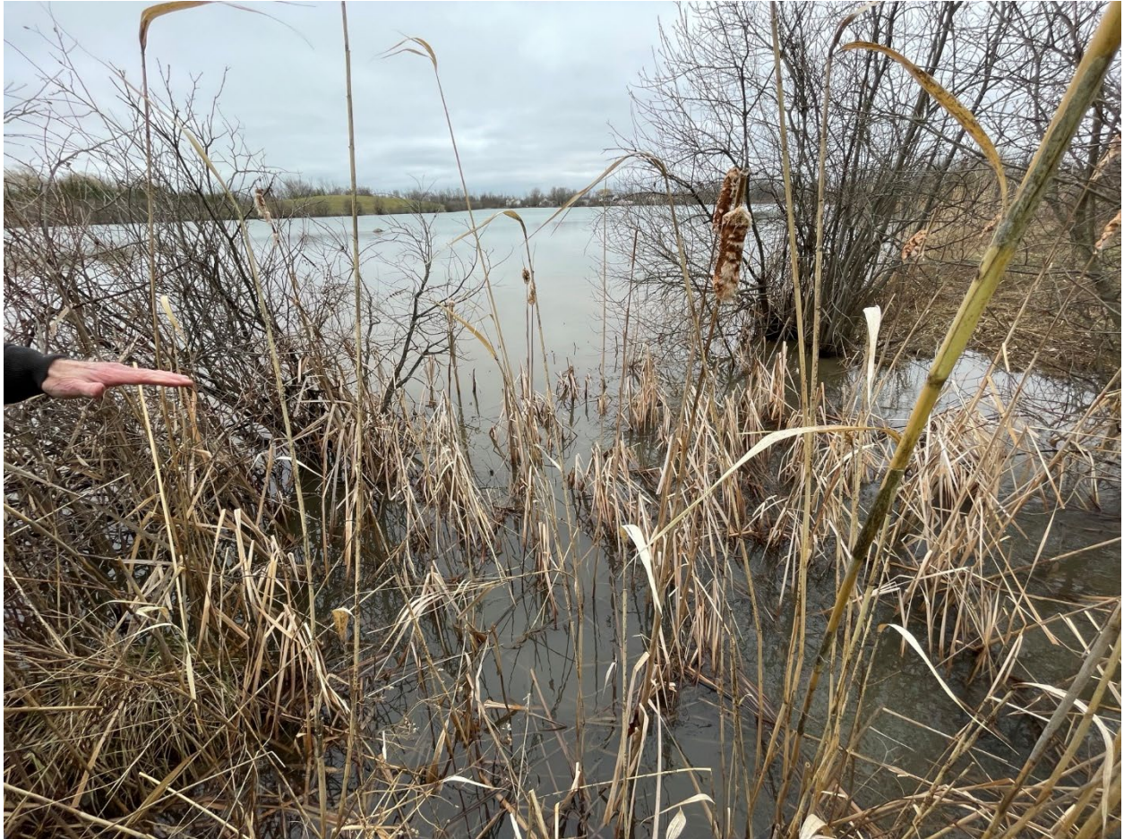
Weir conditions, view facing south.
