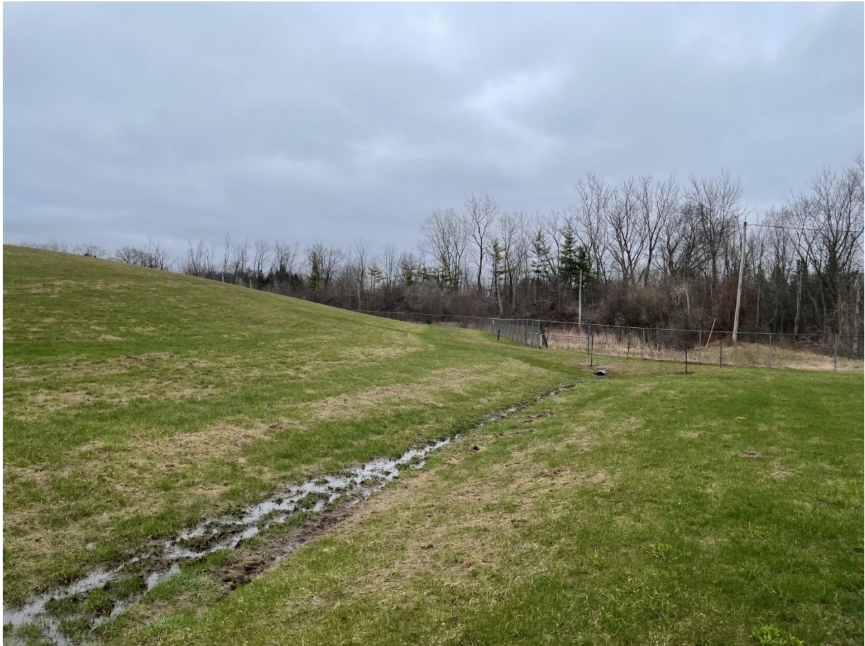
Landfill cap conditions, view facing south/southeast.
