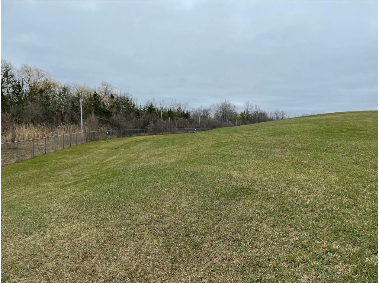
Landfill cap conditions, view facing southwest.
