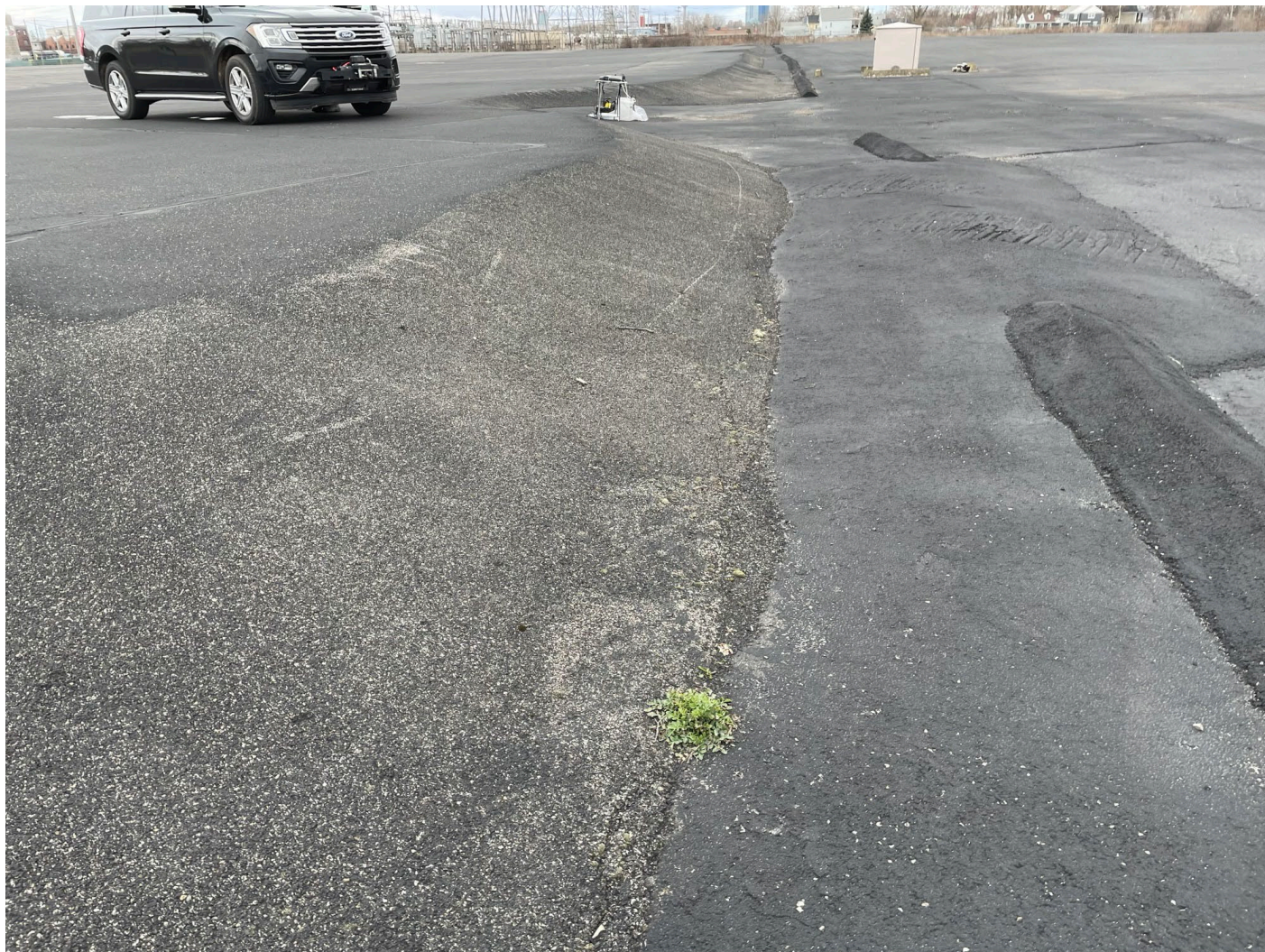
Asphalt cover with minor vegetation growth through cracks.
