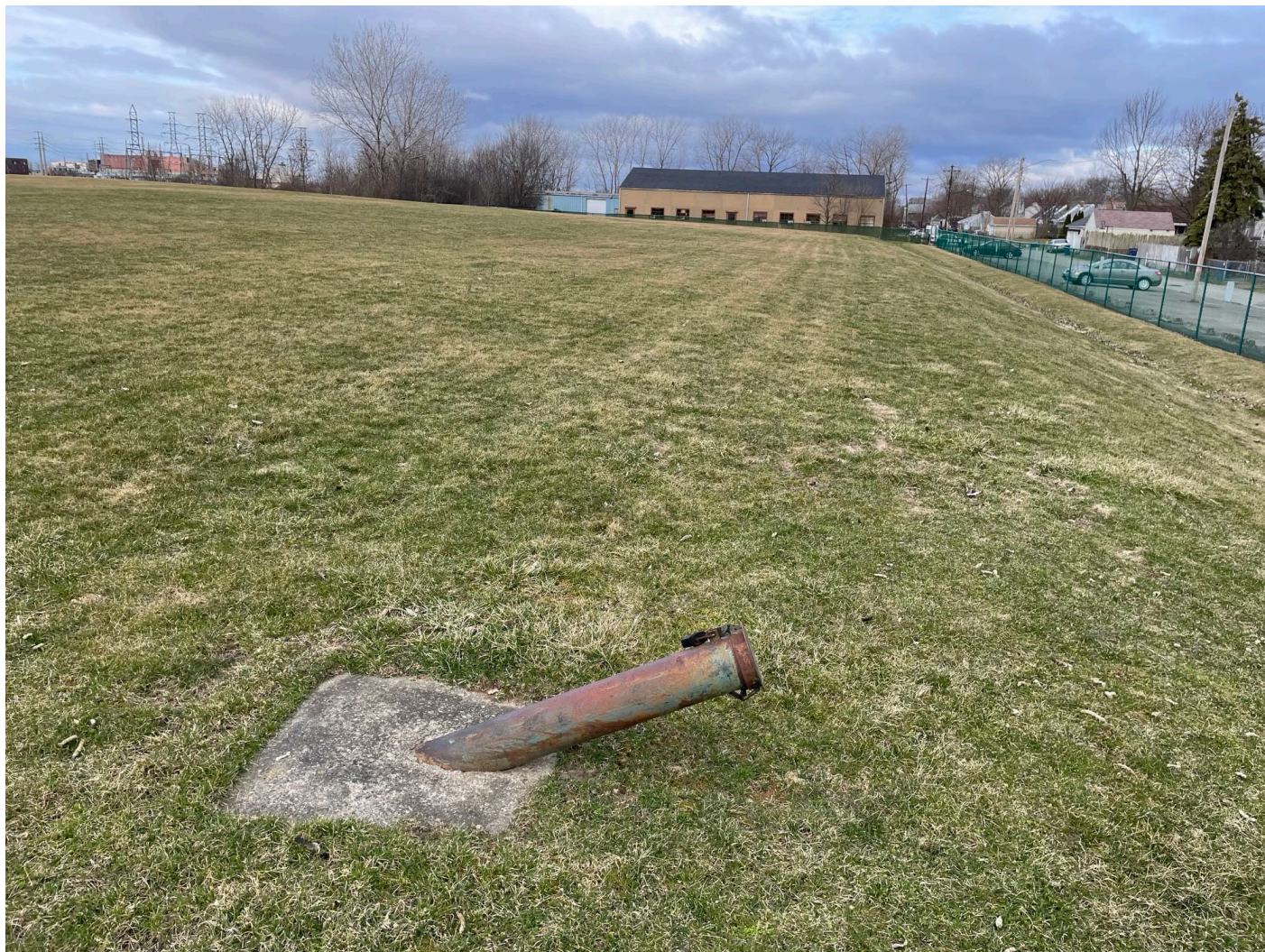
LCRS cleanout pipe/northern vegetative cover facing W.
