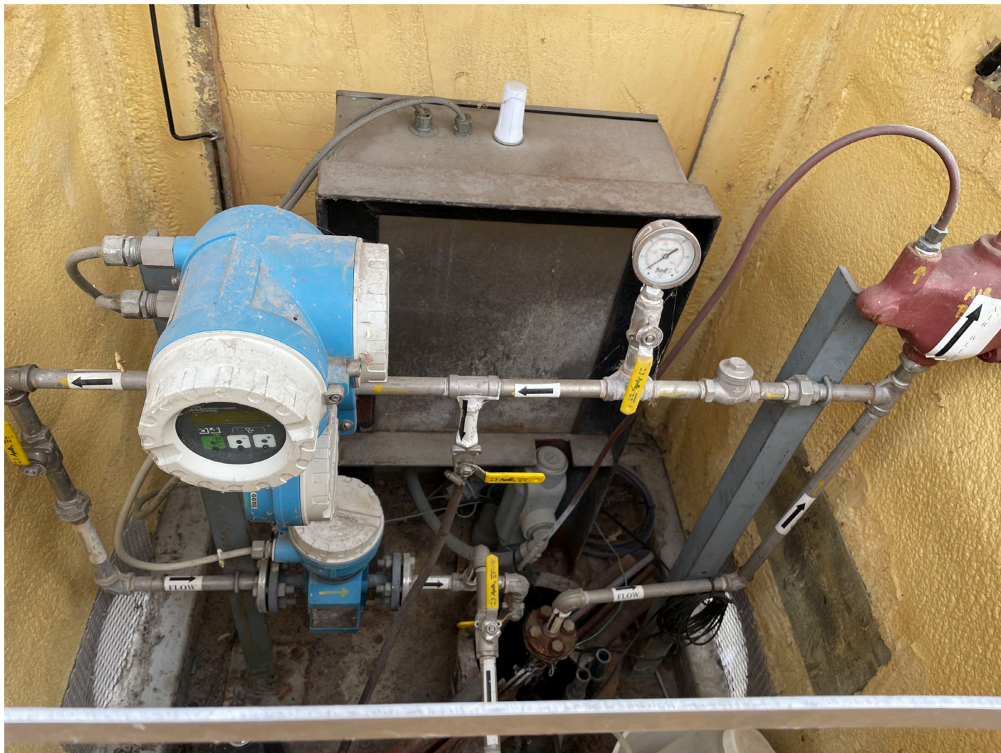
LCRS sumps/piping/flow meter.
