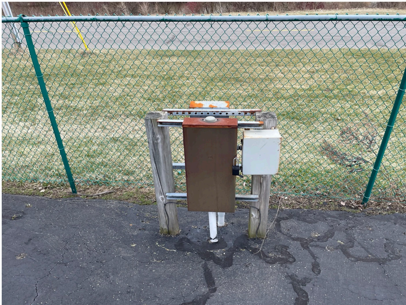
Electric panel/control box for LCRS.
