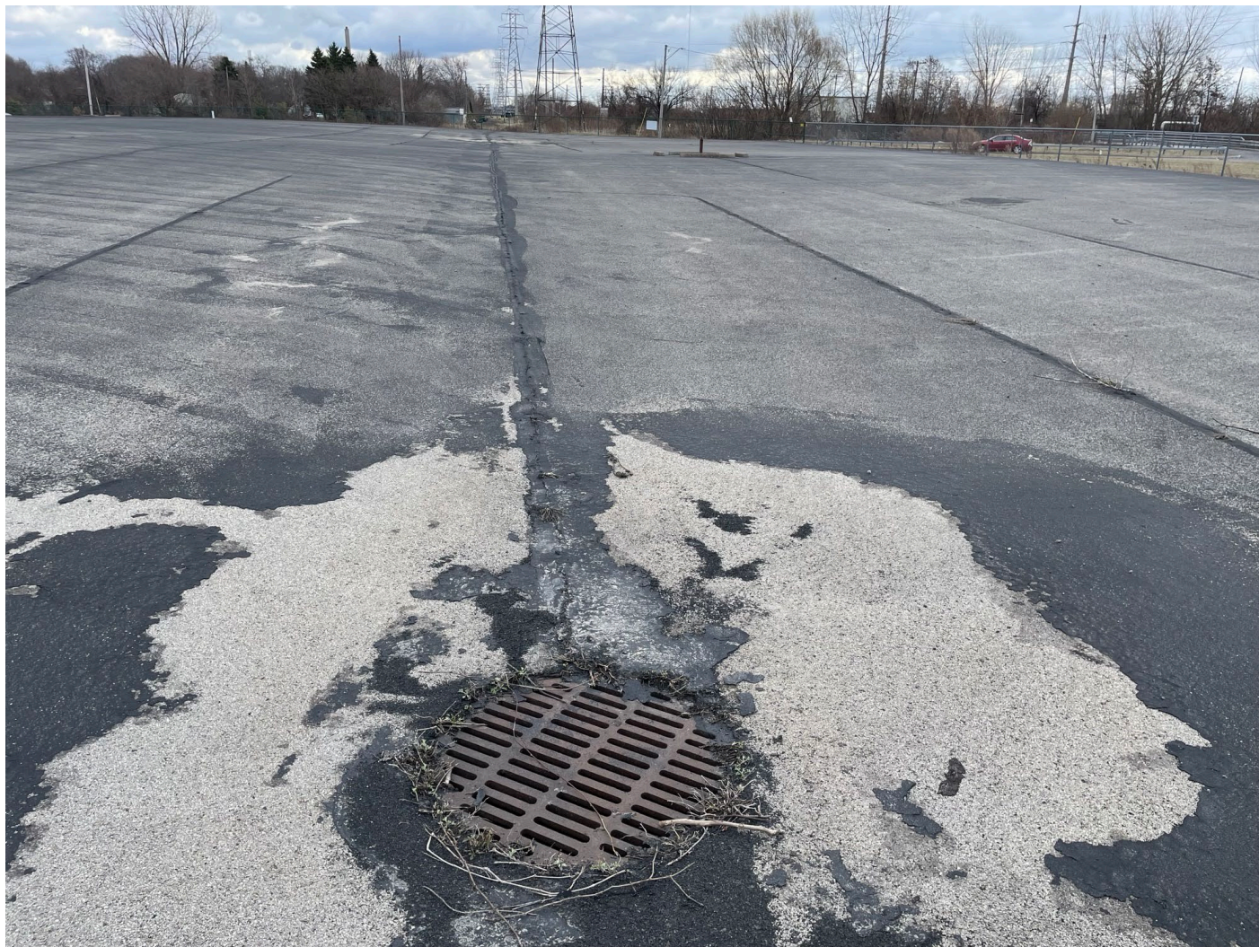
Drop inlet, typical.
