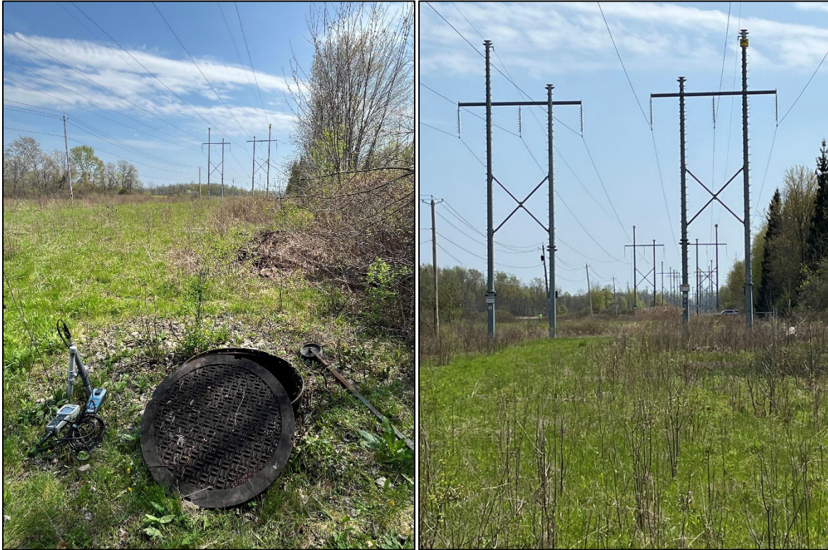
Southward views of the utility right of way where the offsite extraction wells are located; EW-2 vault shown in left photo.
