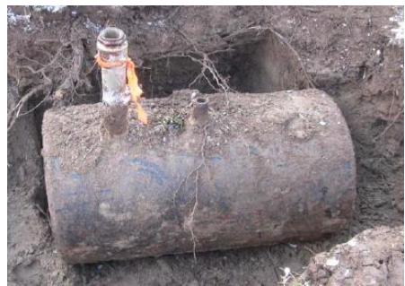
55 gallon UST recovered from this location next to a small concrete foundation. Source: Green Seal Environmental, Inc. (2011)
