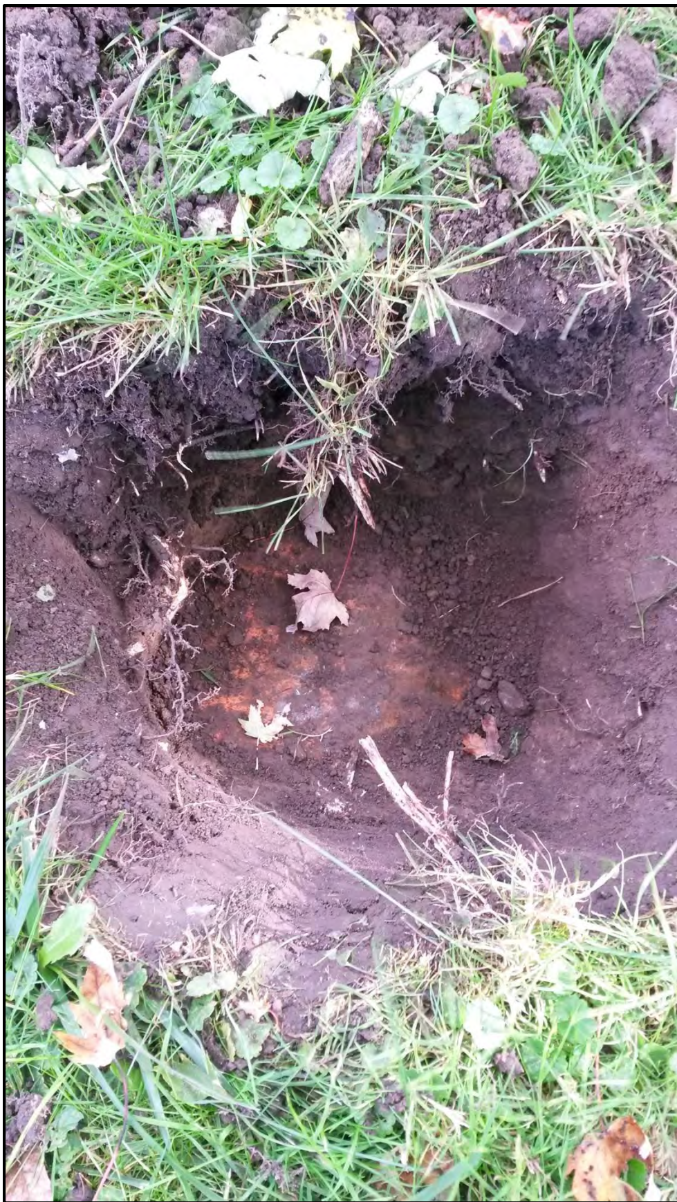
Photo 6: close-up picture of hand dug hole surrounding B-6. Reddish-orange material in hole is the top of the discovered UST.
