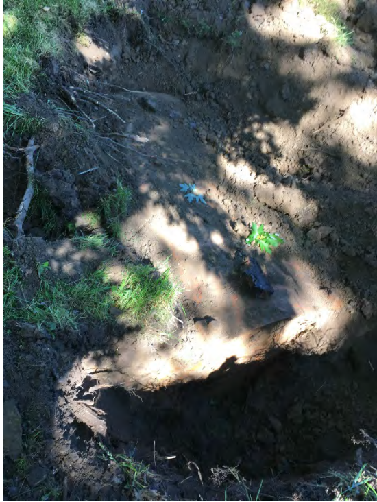
Photo 7 - Tank in Excavation.
