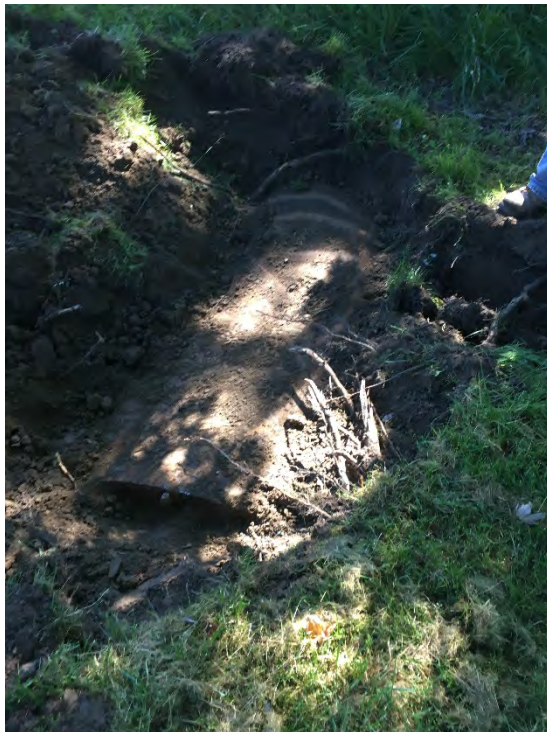
Photo 6 - Home heating oil tank in Excavation.
