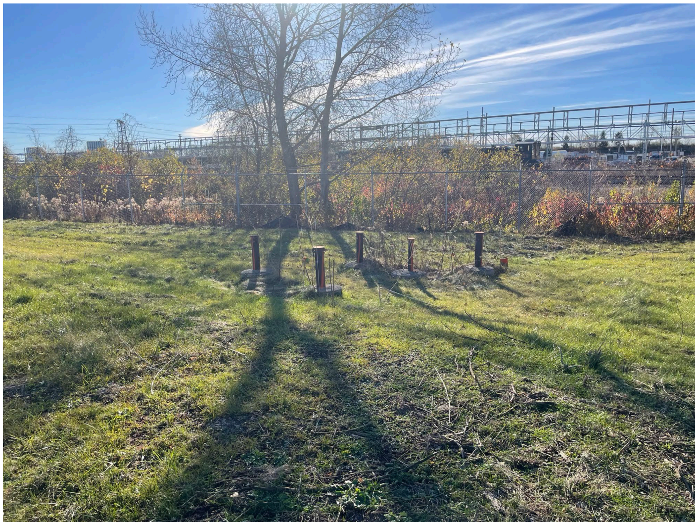
Piezometer/well area in southwest corner.
