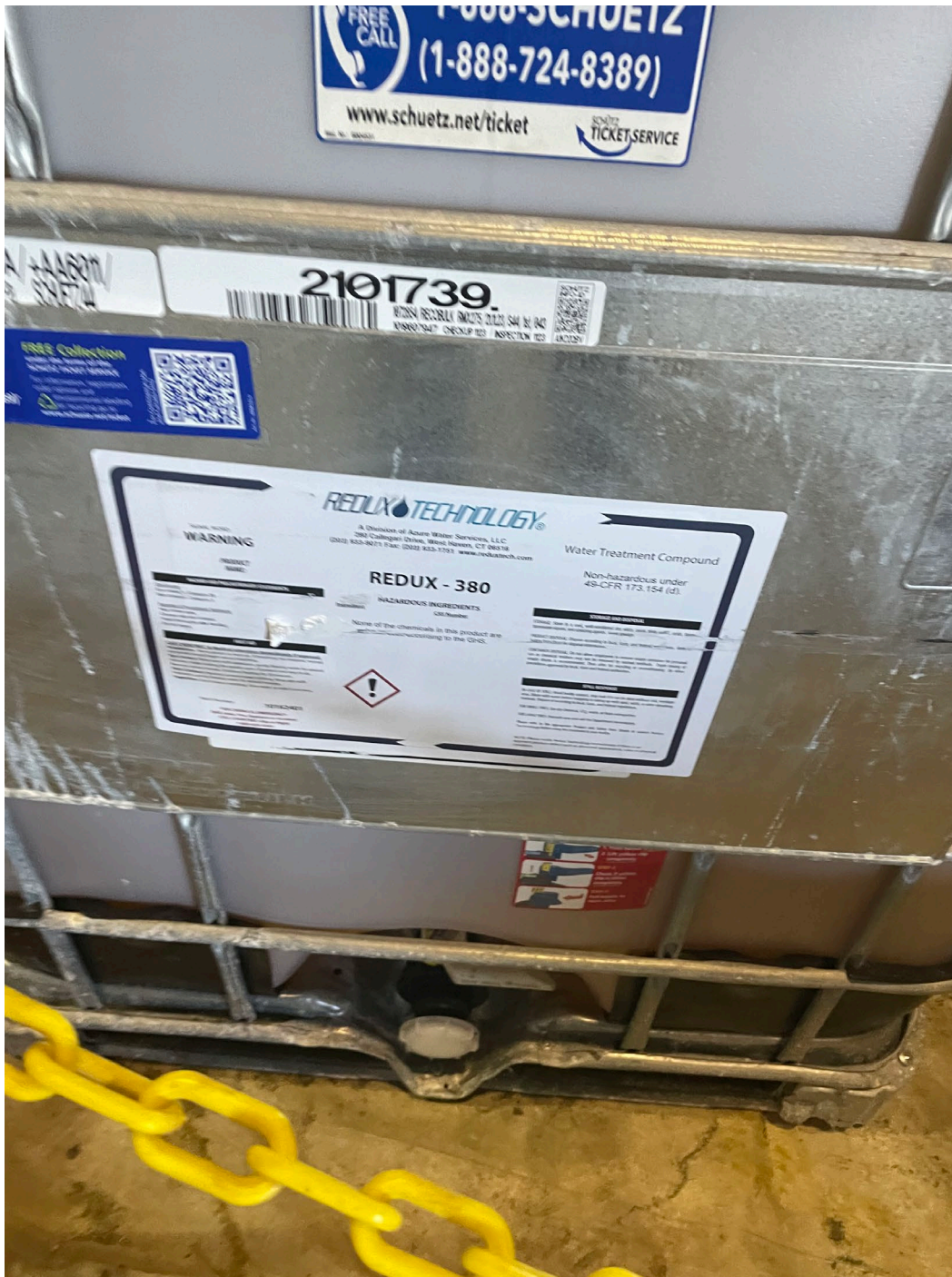
Redux 380 additive to prevent scaling in the carbon vessels.
