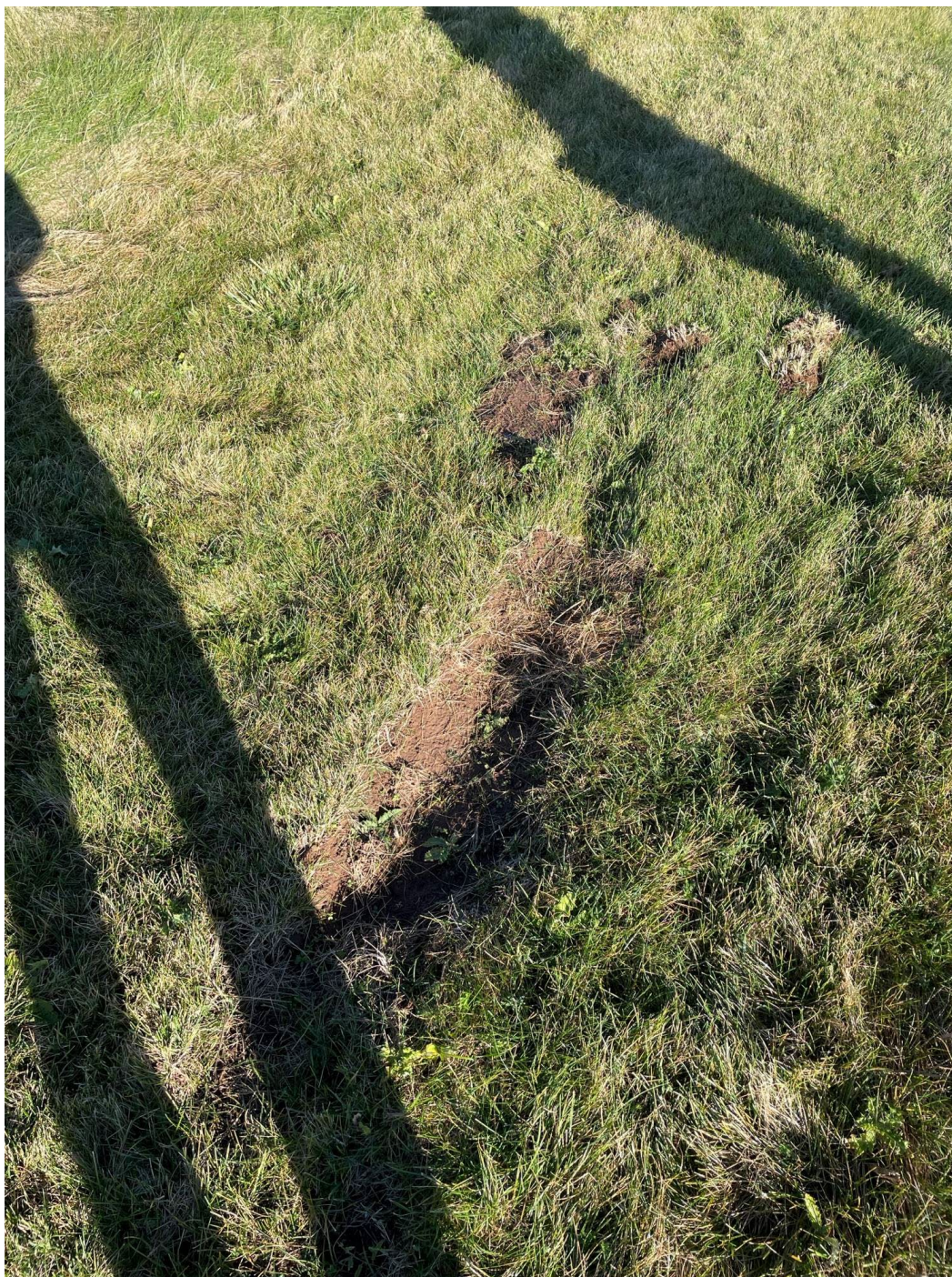
Small rut in NE portion of site cover.
