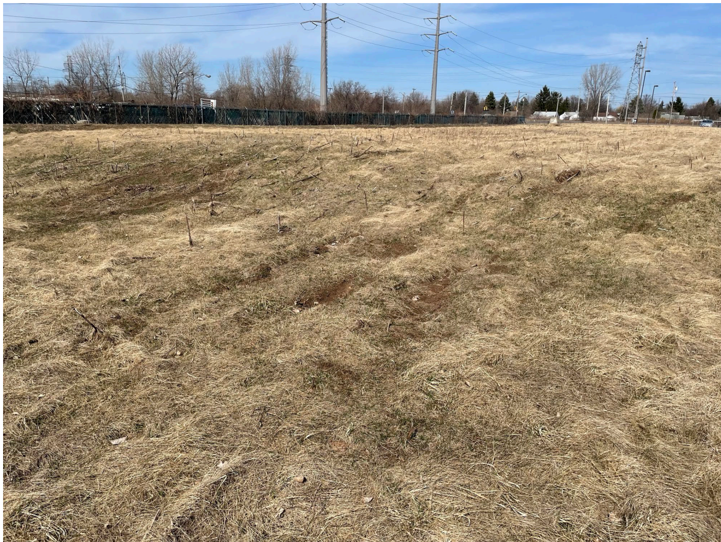
Ruts/bare spots in cover to be monitored for regrowth, view facing N/NW.
