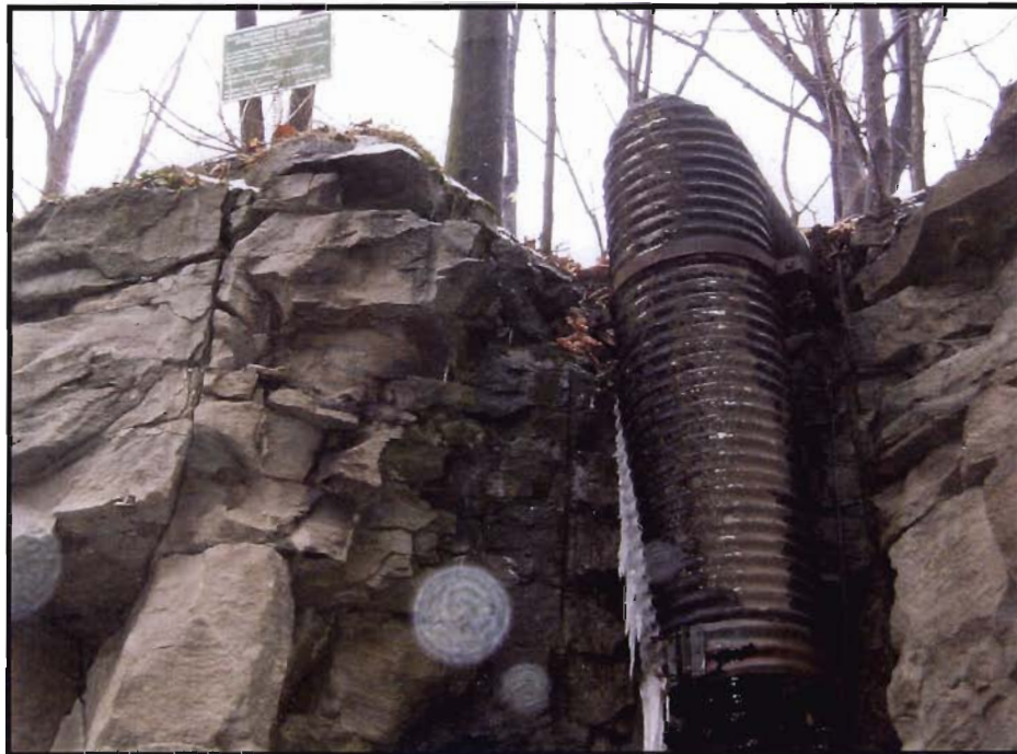
Photograph 7: SPDES Outfall #11 near TS-01. Typical flow of 2-3 gallons per minute.
