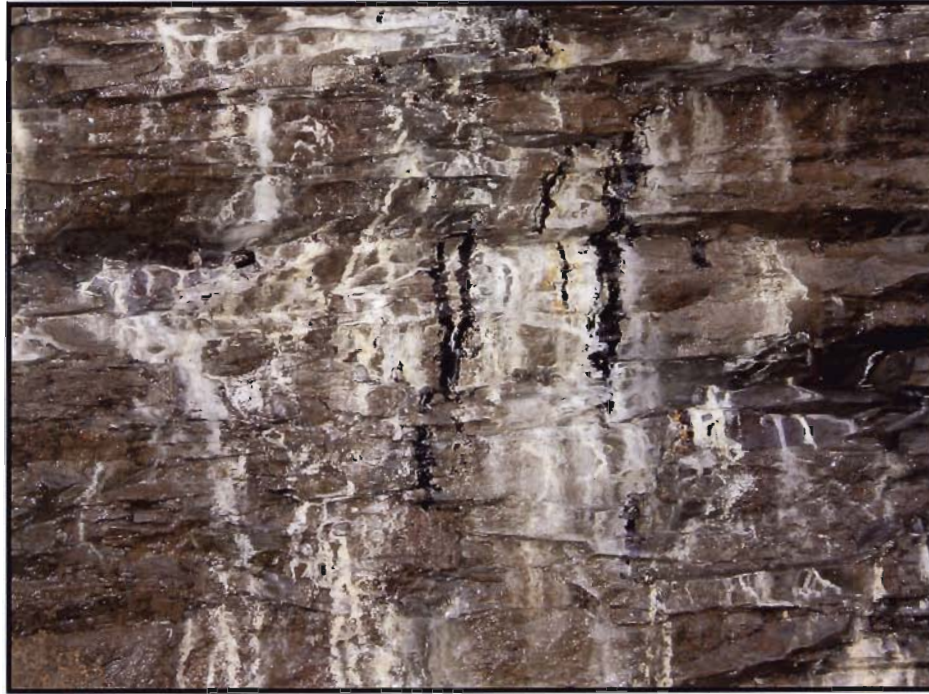
Photograph 6: MGP impacted seeps in the vicinity of TS-10.
