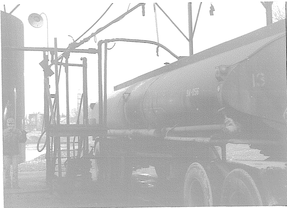
TANK #60 LOADING AREA
