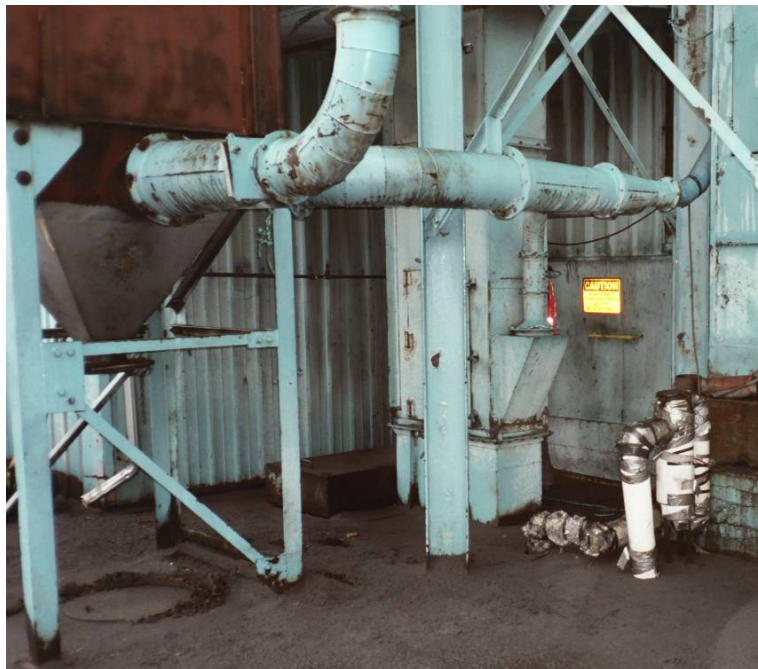
Photograph 6: Vault 4 (sand elevator). The top of the vault is flush with ground level. The vault surrounds the vertical elevator shaft. The PVC sump piping (wrapped in silver tape) is shown on the right.
