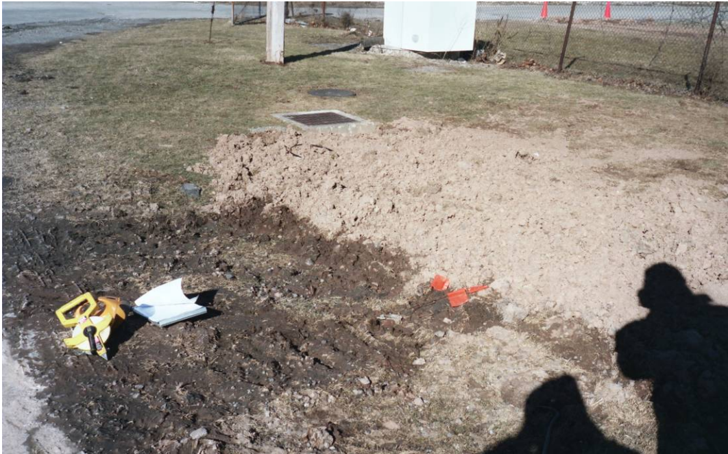
Photograph 1: Area south of CB-10 and MH-3, showing excavated soils from the storm-sewer line replacement by Metaullics in February 2006. Broken sanitary clean-out visible near orange flags. POTW shed in background.
