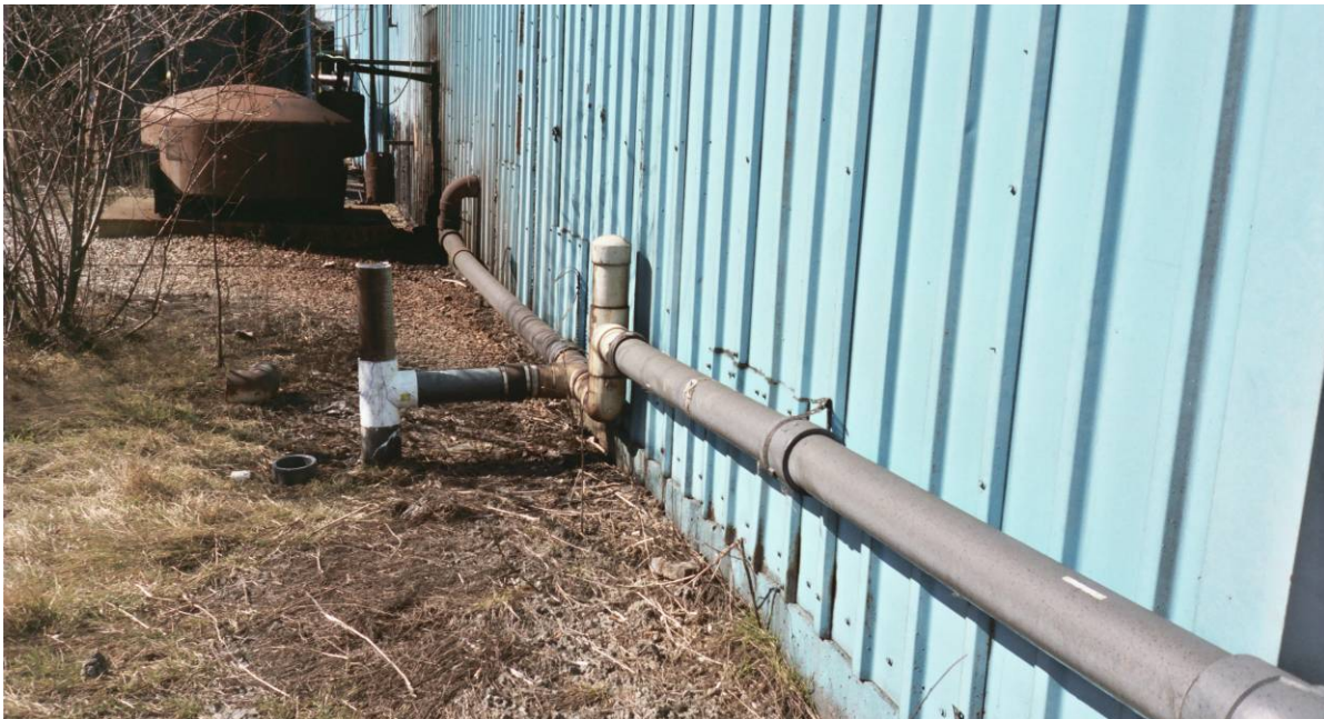
Photograph 2: Pipe D-1 connects to the sanitary sewer. Water from process cooling, Sump 2, and Sump 3 is pumped into D-1.
