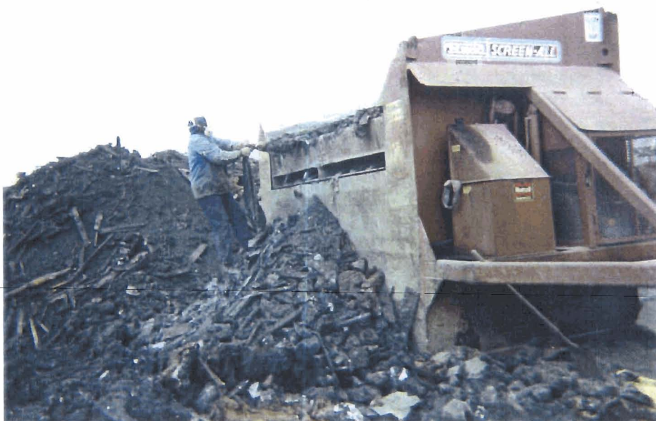
LABORER REMOVING DEBRIS FROM GRID
