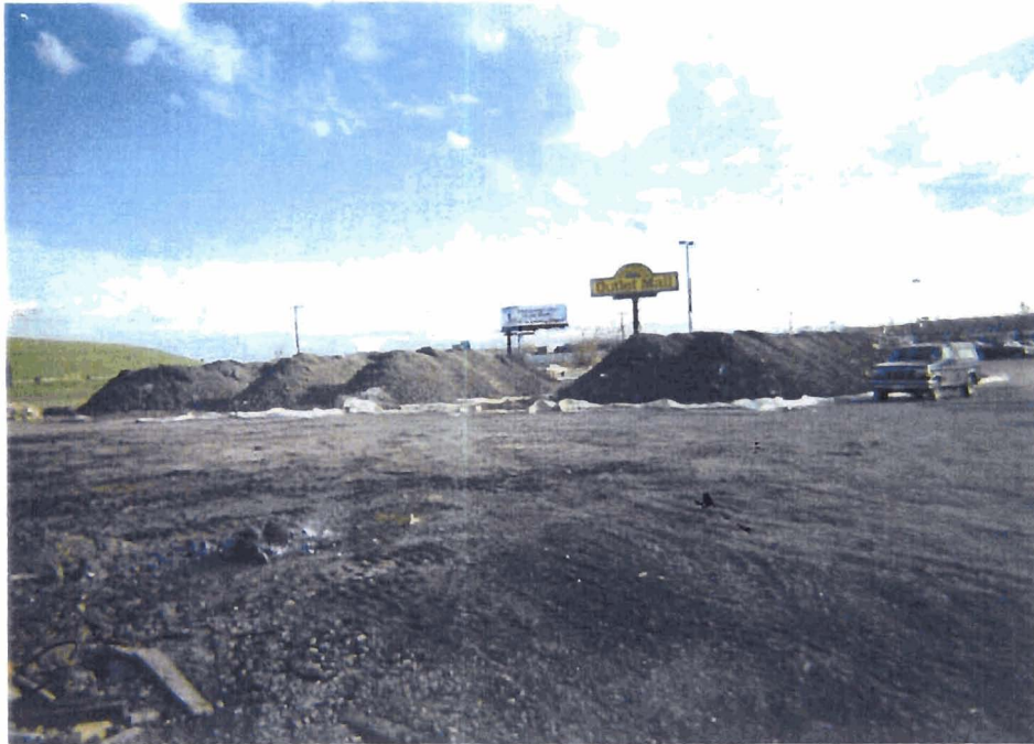
FINAL LANDFARM WINDROWS OF SCREENED SOIL
